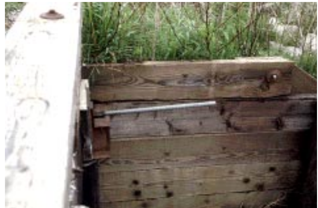
Figure 21—Stressing bar angles upward at southeast corner of Decatur bridge.
