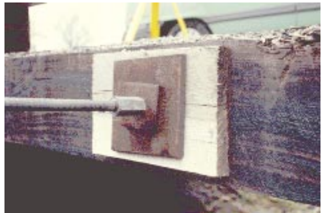
Figure 4—Details of the Dean (top), Hibbsville (middle), and Decatur (bottom) discrete plate anchorage configurations.
