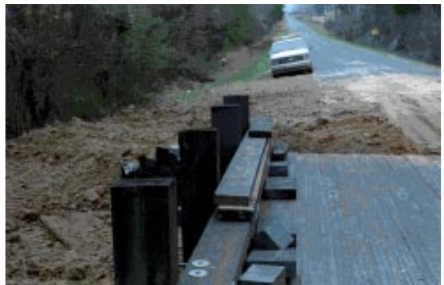
**Figure 9—Attachment of bridge curb and rail system following the second bar tensioning.**
