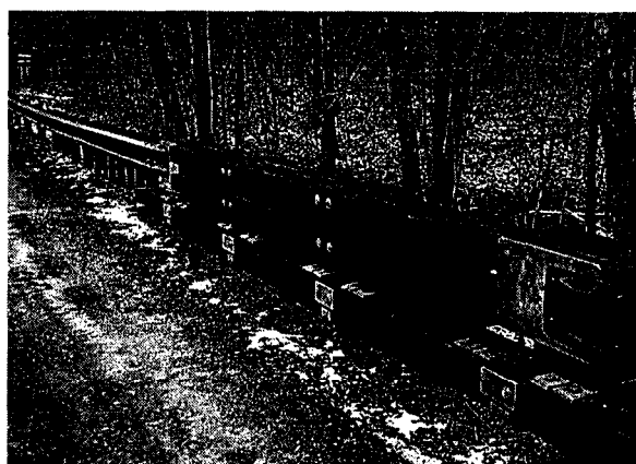
Figure 4—Yellow-poplar glulam bridge railing
