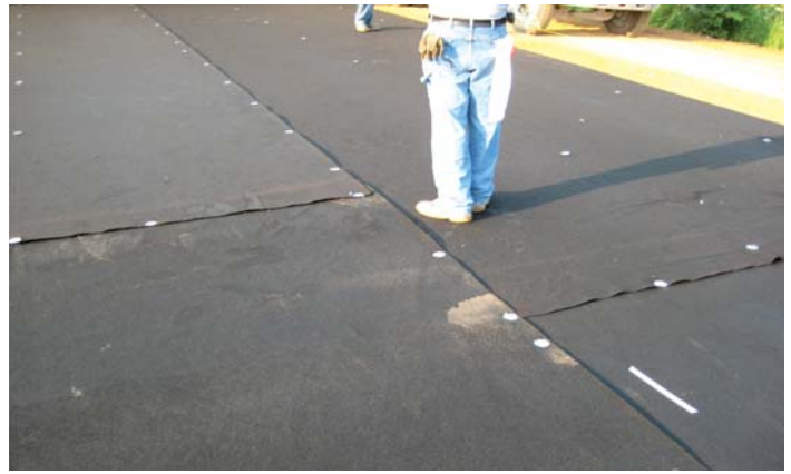
Figure 5. Overlap of nonwoven geotextile material sections
