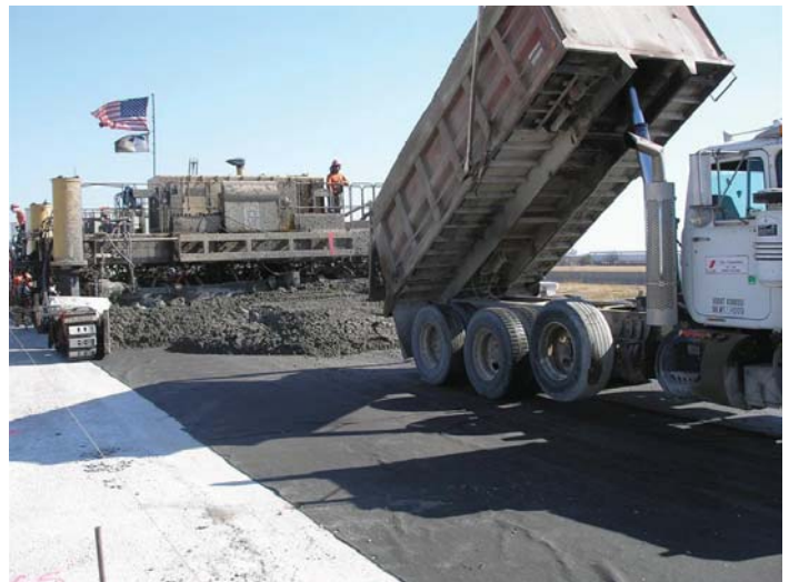
Figure 7. Paving on top of nonwoven geotextile materials
