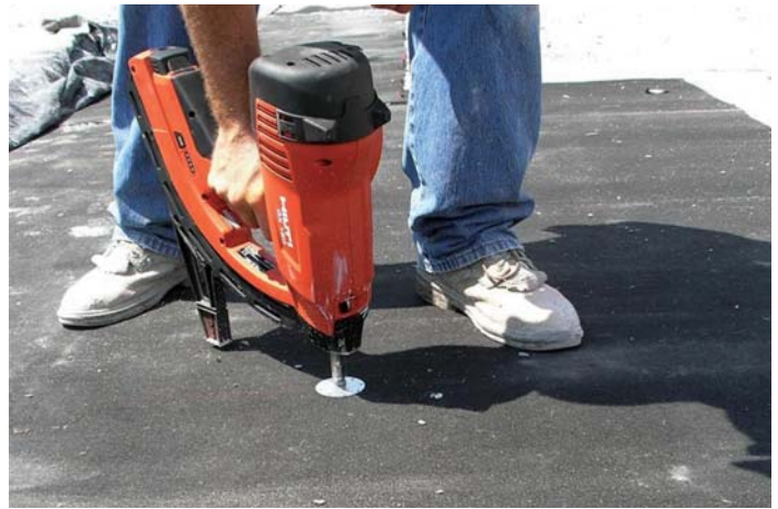
Figure 6. Fastening nonwoven geotextile fabric to existing concrete pavement
