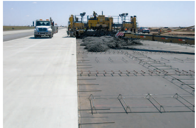
Figure 30. Texas Lubbock Preston Smith International Airport– During overlay placement
