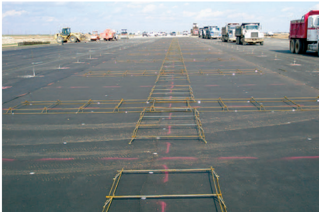
Figure 30. Texas Lubbock Preston Smith International Airport– During overlay placement
