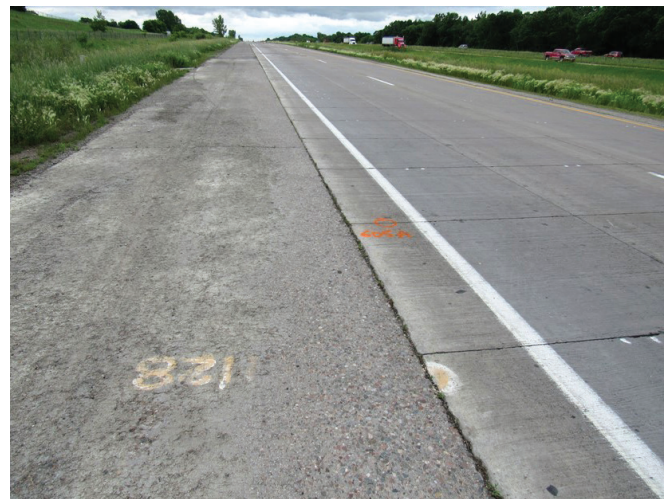
Figure 34. MnROAD Test Section 605 – 5 in. UBOL on standard fabric – June 2016
