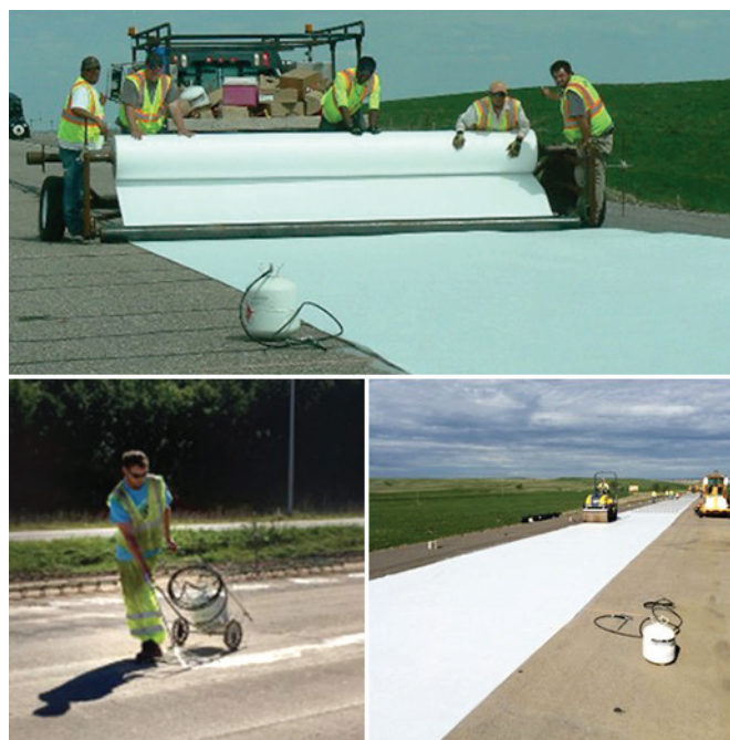
Figure 12. Securing geotextile with spray adhesive
