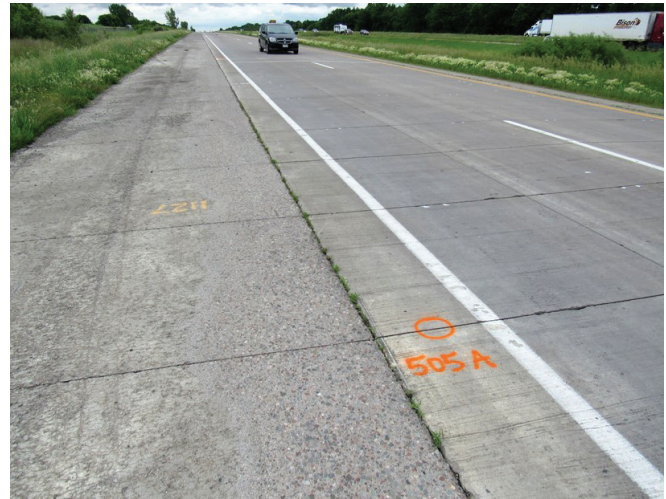
Figure 33. MnROAD Test Section 505 – 5 in. UBOL on standard fabric – June 2016
