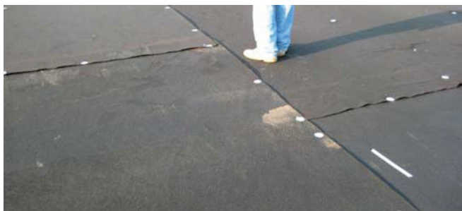
Figure 10. Overlap of nonwoven geotextile material section
