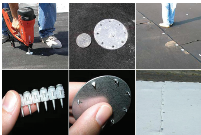
Figure 11. Securing geotextile (pins/nails) with washer
