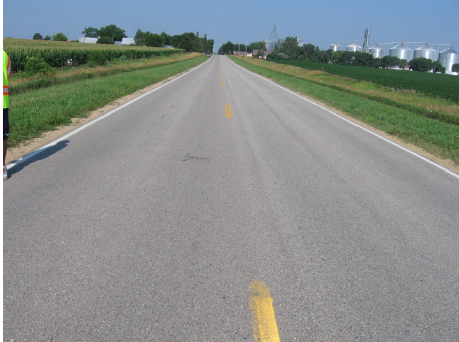
Figure C.18. Overall Pavement Condition on C23 in Franklin County, IA (I.D. No. 26): Rubbblization
