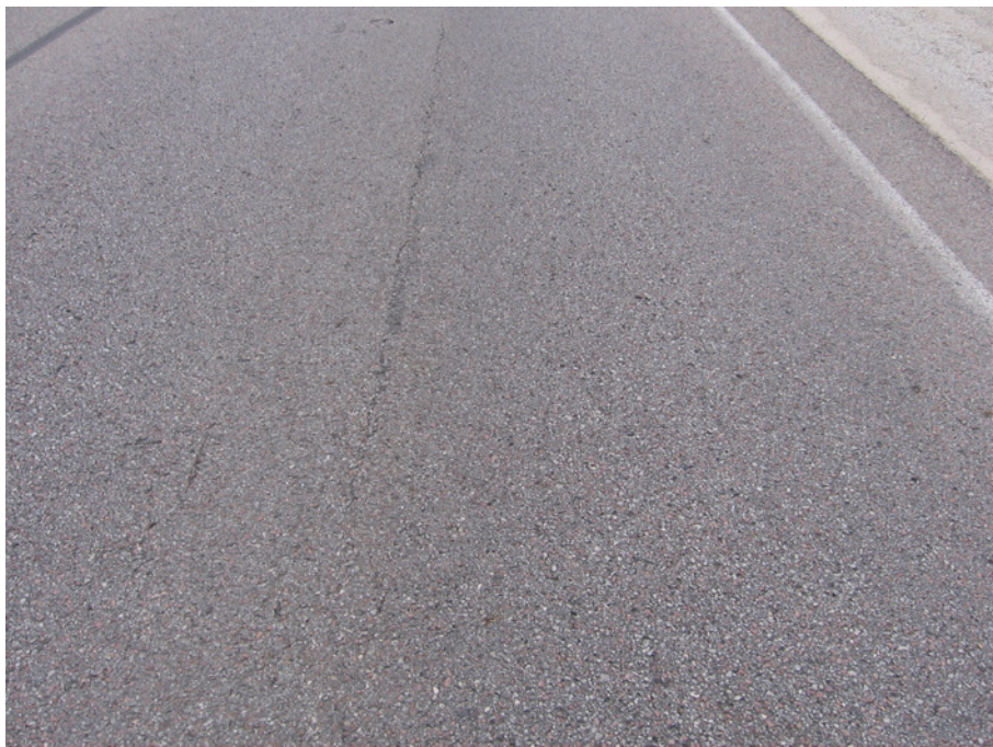
Figure C.30. Longitudinal Crack on IA141 in Polk County, IA (I.D. No. 33-1): Rubblization
