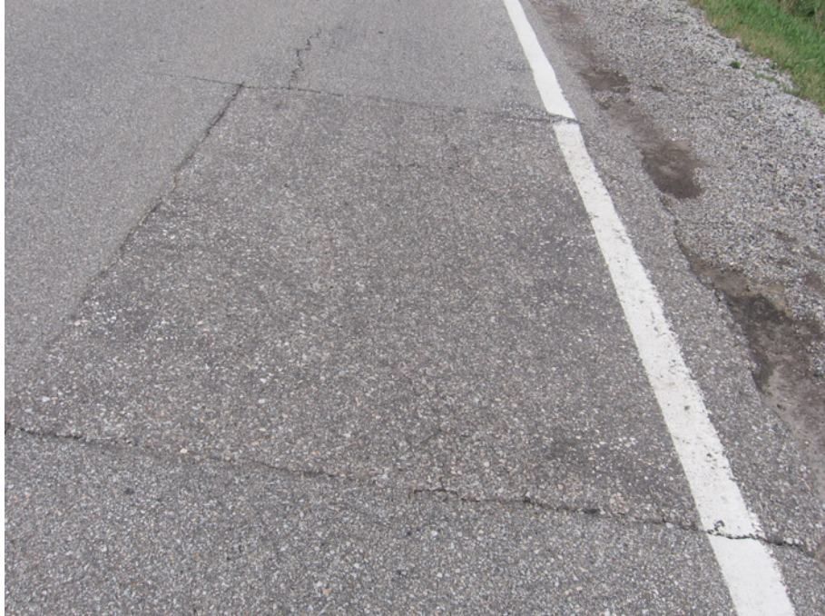
Figure C.10. Block Crack on V43 in Black Hawk County, IA (I.D. No. 13): Rubblization
