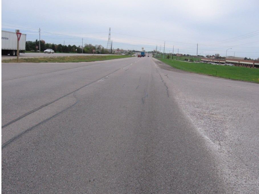
Figure C.27. Overall Pavement Condition on IA141 in Polk County, IA (I.D. No. 33-1): Rubblization
