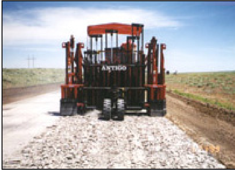
Figure 2. Multi-Head Breaker (Antigo Construction, Inc.)
