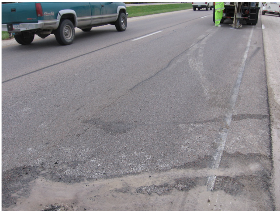
Figure C.34. Longitudinal Crack on IA141 in Polk County, IA (I.D. No. 33-2): Rubblization
