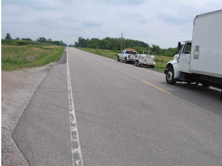
Figure C.3. Pavement Condition at location B (Middle) of D16 in Black Hawk County, IA (I.D. No. 12): Rubblization
