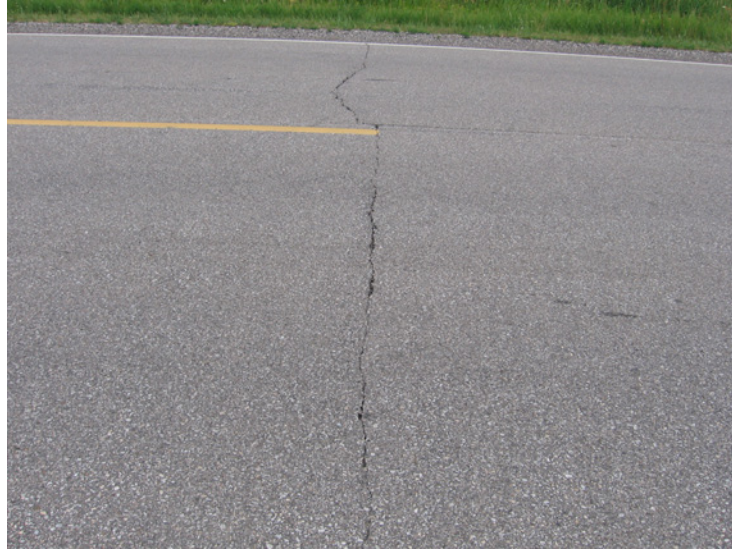
Figure 13. Picture of low-temperature cracking on HMA-overlaid rubblized PCC (I.D. No. 12: D16 in Blackhawk County)
