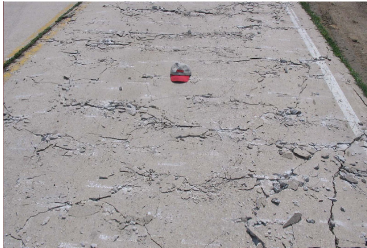
Figure 6. Modified Rubblization Method proposed by Antigo (Jansen, 2006)
