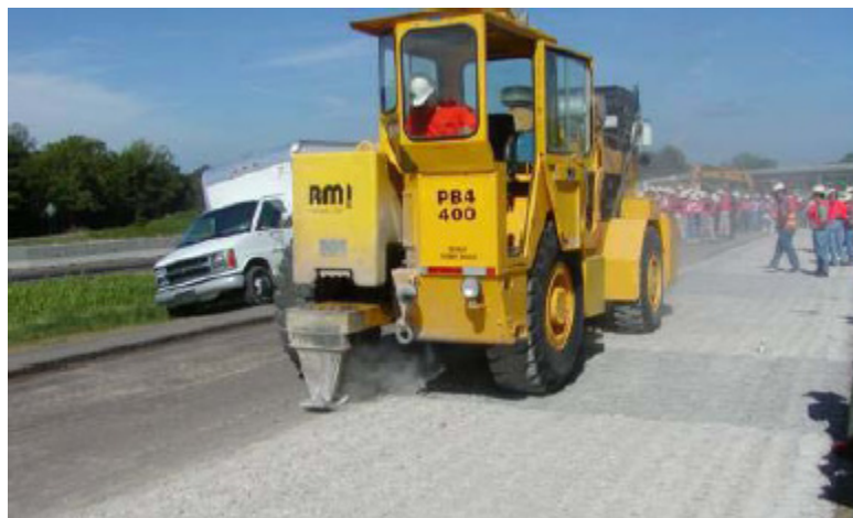
Figure 1. Resonant Pavement Breaker (Resonant Machines, Inc.)
