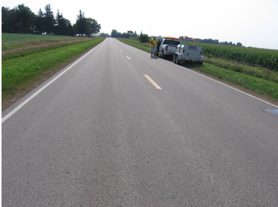
Figure C.20. Pavement Condition on B (Middle) of C23 in Franklin County, IA (I.D. No. 26): Rubblization
