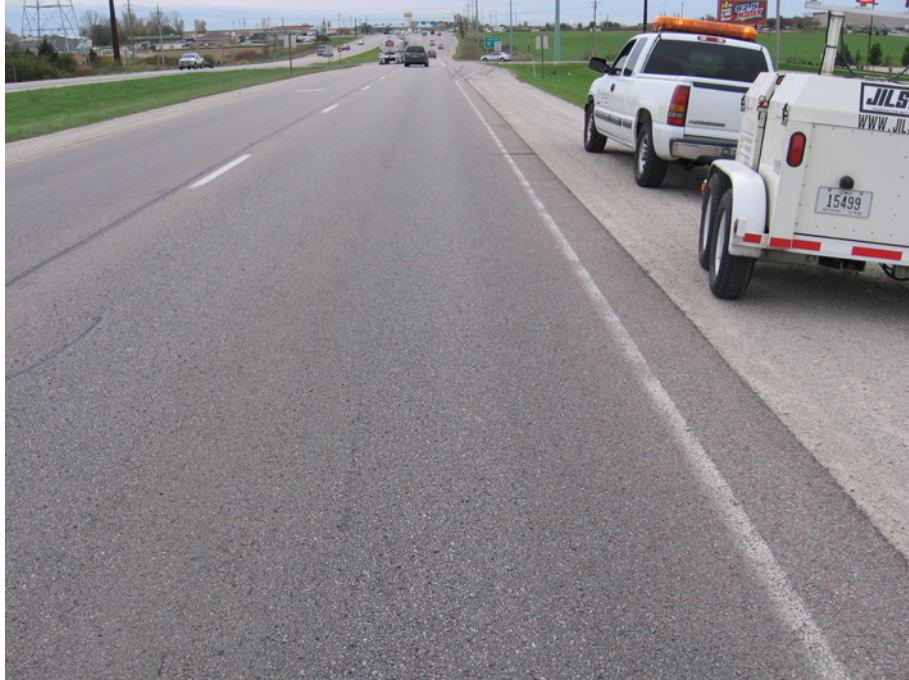
Figure C.31. Overall Pavement Condition on IA141 in Polk County, IA (I.D. No. 33-2): Rubblelization
