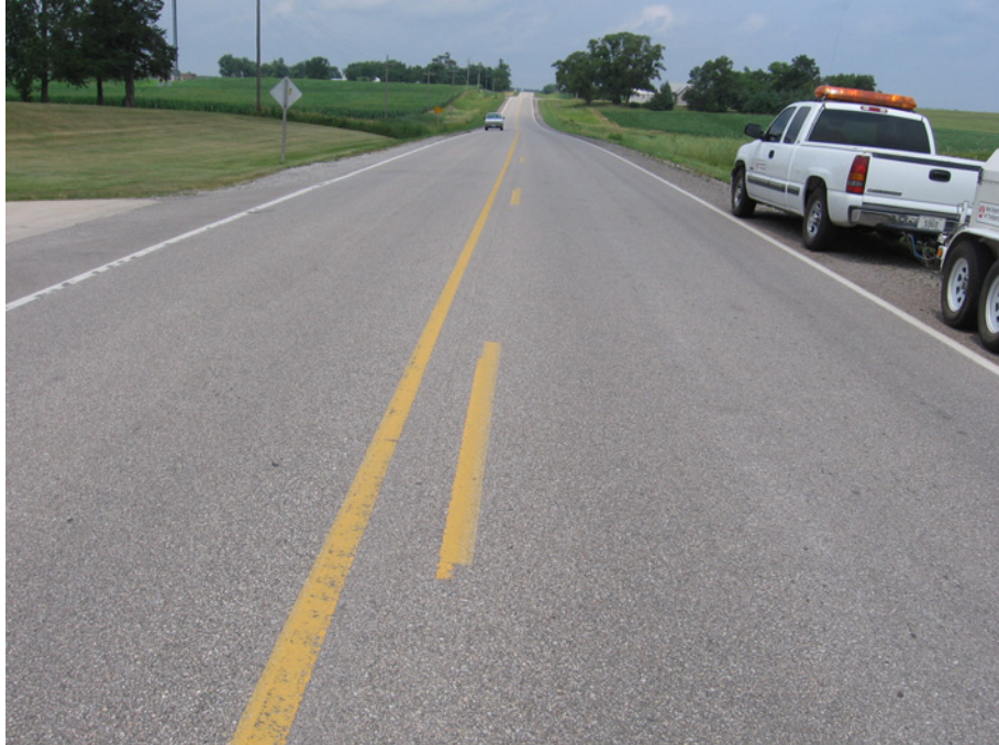
Figure C.6. Overall Pavement Condition on V43 in Black Hawk County, IA (I.D. No. 13): Rubbblization
