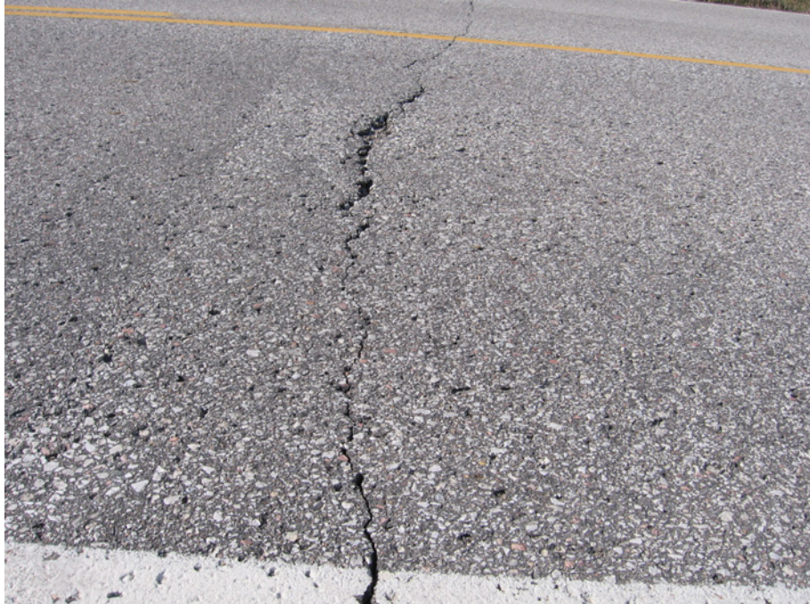
Figure C.26. Low Temperature Crack on L55 in Mills County, IA (I.D. No. 32): Rubblization
