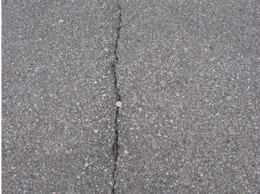
Figure C.5. Low Temperature Crack on D16 in Black Hawk County, IA (I.D. No. 12): Rubbblization
