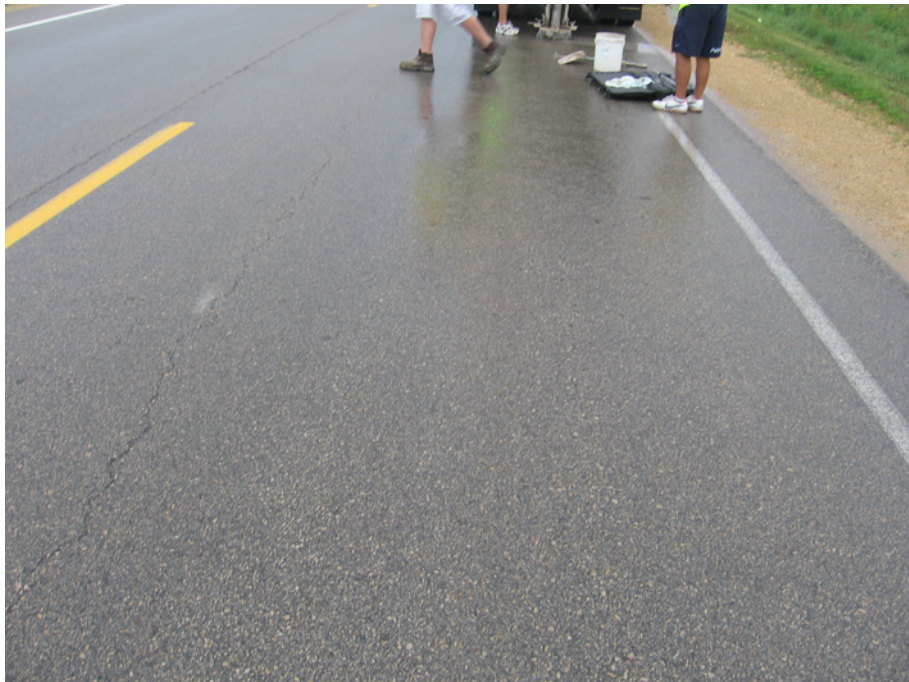
Figure C.16. Longitudinal Crack on IA3 in Delaware County, IA (I.D. No. 21): Rubblization
