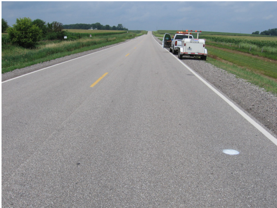
Figure C.8. Pavement Condition on B (Middle) of V43 in Black Hawk County, IA (I.D. No. 13): Rubblization
