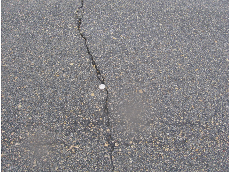
Figure C.17. Low Temperature Crack on IA3 in Delaware County, IA (I.D. No. 21): Rubbblization
