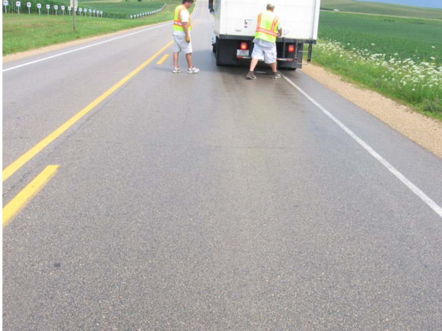
Figure C.15. Pavement Condition on C (End) of IA3 in Delaware County, IA (I.D. No. 21): Rubblization
