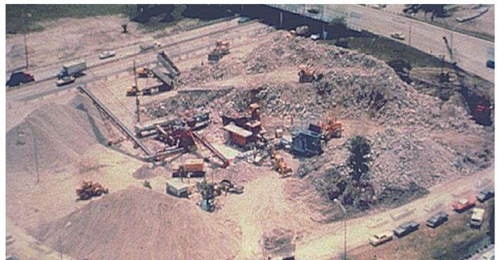
Figure 4. Concrete recycling operation set up inside of Edens Expressway cloverleaf interchange (photo from NHI 1998)
