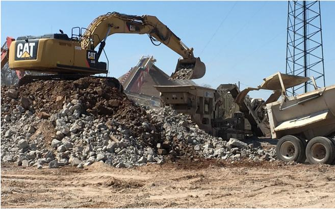
Figure 4. On-site crushing operation (photo courtesy of Gary Fick, Trinity Construction Management Services)
