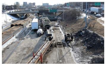
Dwayne Stenlund/MnDOT Figure 1. Well-implemented on-site material crushing program in urban area
