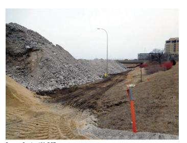
Dwayne Stenlund/MnDOT Figure 5. Concrete stockpiles set inside of roadway depression with stormwater inlets taken off line
