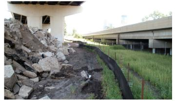
Dwayne Stenlund/MnDOT Figure 2. Demolished material stockpiled beneath bridge prior to crushing with silt fence and vegetative buffer
