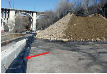
Dwayne Stenlund/MnDOT Figure 6. High-performance perimeter control using concrete blocks wrapped in geotextile fabric
