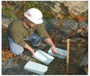
Copyright @ 2016 Hydrograss Figure 10. Floc log tied to wooden stake in outflow path
