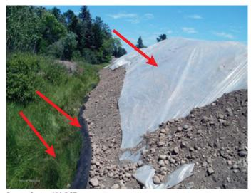
Dwayne Stenlund/MnDOT Figure 8. RCA stockpile tarped with plastic and bounded by perimeter berm of wrapped RCA
