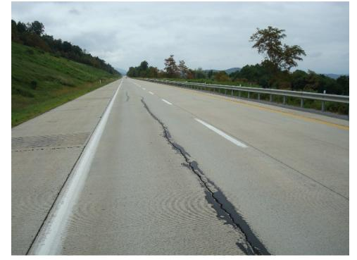
Figure 6.14 Longitudinal crack in over-failed strand in post-tensioned concrete pavement on Pennsylvania I-99
