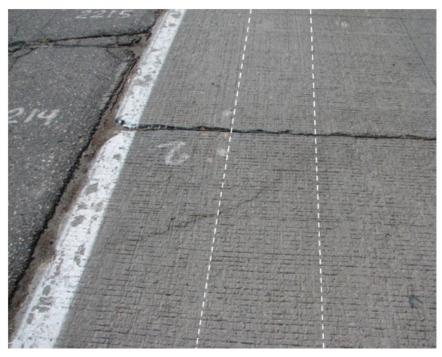
c. Low-severity corner crack at exterior location with evidence of pumping along lane-shoulder joint Julie Vandenbossche, University of Pittsburgh
