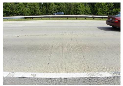
Figure 13.2 Closely spaced transverse cracks in 25-year-old CRCP
