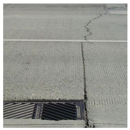
b. Sympathy crack from joint aligning with catch basin Jeff Uhlmeyer, Washington State DOT
