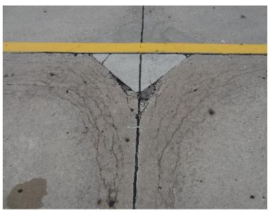
Figure 4.3 Staining accompanying D-cracking at joints
