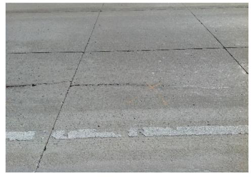
Figure 18.2 Common UBCOC-specific distresses
