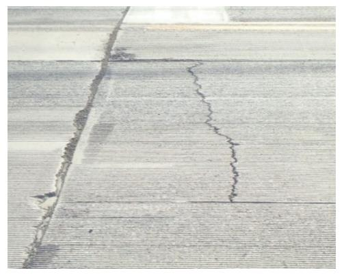
c. Reflective crack over unrepaired transverse crack near transition  $${\rm Mark\ Snyder,\ PERC}$$
