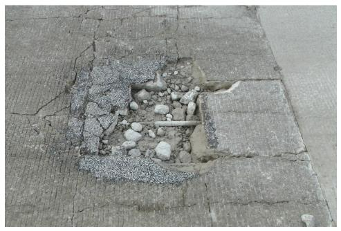
Figure 13.4 Insufficient depth of cover
