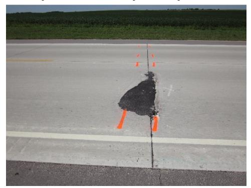
Figure 17.10 Transverse cracking due to misaligned dowels\*
