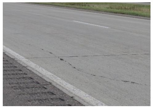
**b. Longitudinal cracking in wheel path in UBCOC** Tom Burnham, Minnesota DOT
