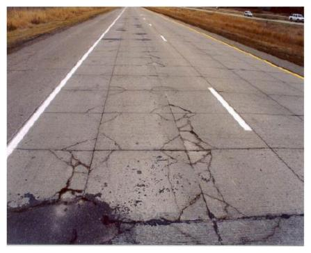
b. Corner cracking at interior locations (late stages), leading to development of shattered panels Tom Burnham, Minnesota DOT
