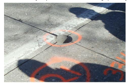
Figure 7.8 Small corner crack, possibly due to infiltration of mortar during adjacent lane placement
