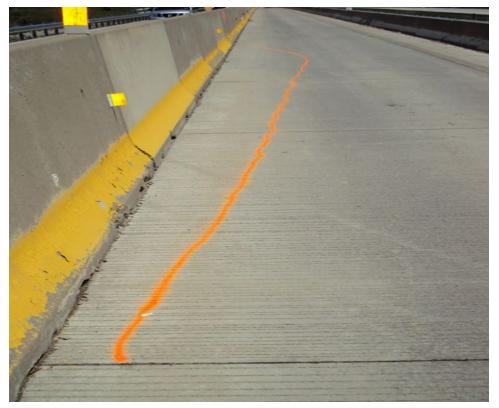
e. Longitudinal crack along centerline joint with possible late sawing Mark B. Snyder, used with permission
