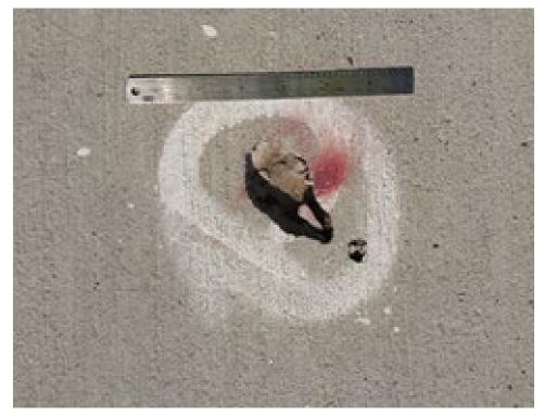
Figure 2.2 Void created by clay ball at the concrete surface
