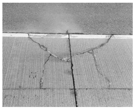
d. Well-developed corner cracks at exterior location with evidence of pumping along lane-shoulder joint and secondary transverse cracking
