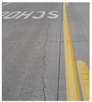
c. Longitudinal cracking due to late sawing Dan DeGraaf, Michigan Concrete Association
