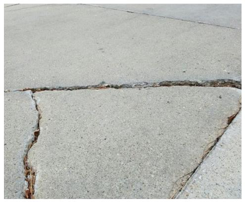
Figure 12.12 Localized settlement due to subgrade movement (consolidation)
