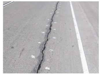
**b. Cross-stitched longitudinal crack** Smith et al. 2014
