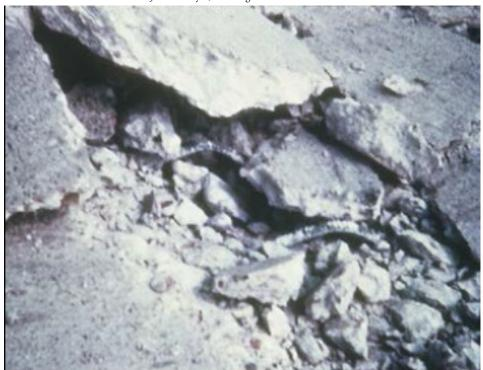
c. Blowup in CRCP showing exposed steel Miller and Bellinger 2014
