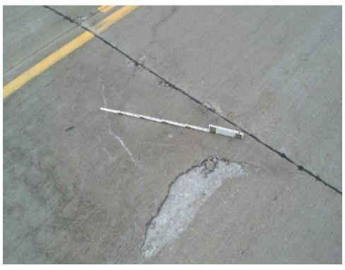
Figure 3.1 Delamination in concrete pavements
