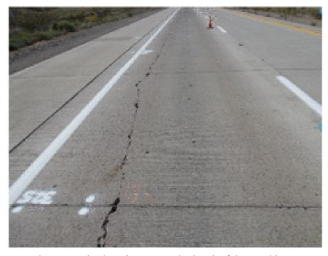
**b. Longitudinal crack in outer wheel path of the travel lane** Long Term Pavement Performance Program (LTPP)
