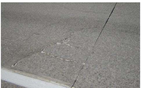
Figure 10.6 Delamination cracking from excessive upward curvature
