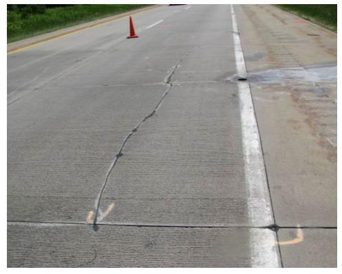
e. Longitudinal crack due to overlay fatigue after debonding Randy Riley, Illinois Chapter, Inc. – American Concrete Pavement Association
