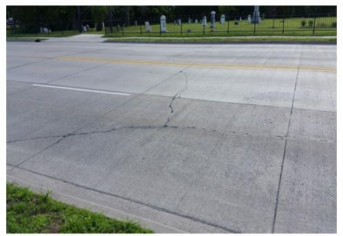
Figure 5.2 Transverse cracking caused by volumetric changes
