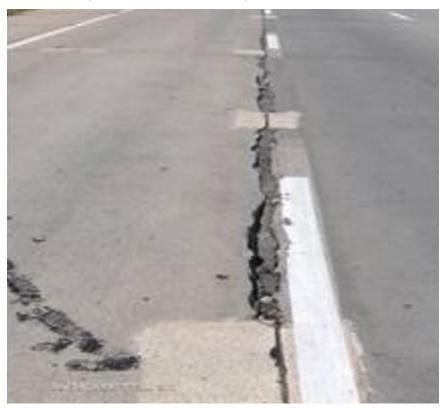
Figure 8.1 Common spalling of joints and cracks
