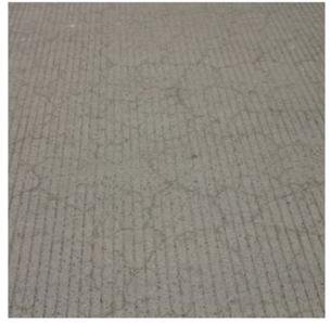
Minor deformities or imperfections that are limited to the surface of a concrete pavement are often referred to as surface defects. These distresses typically do not significantly detract from the structural integrity of the pavement but can have an impact on its functional performance and its aesthetic appeal.
