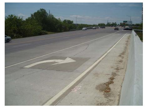
a. Longitudinal cracking due to nonuniform support John Donahue, Missouri DOT
