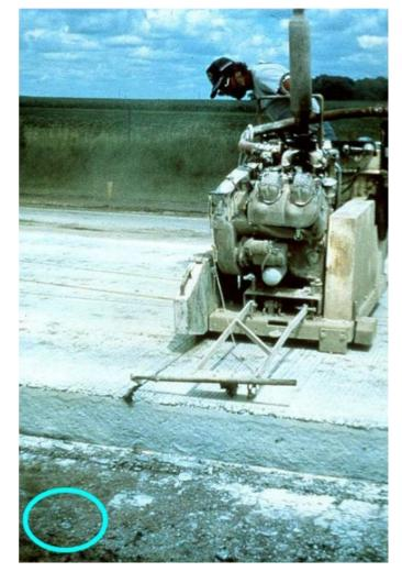
Figure 16.8 Use of nail and washer in shoulder (see circled area) to mark existing joint line prior to overlay placement and joint sawing
