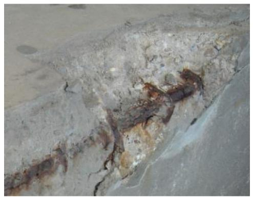
b. Close-up view of corrosion of reinforcing steel causing spalling John Donahue, Missouri DOT
