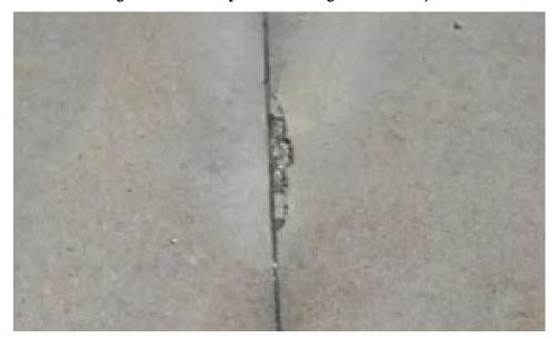
Figure 8.10 Incompressible damage to concrete joint
