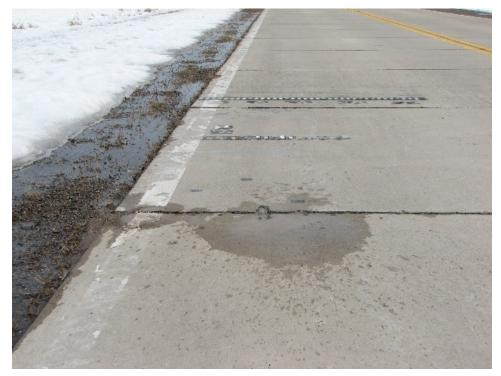
Figure 7.4 Water that has been ejected from a transverse joint under a moving wheel load
