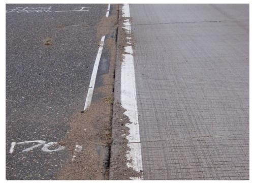
Figure 7.6 Pumped foundation material along longitudinal joint at MnROAD Cell 40
