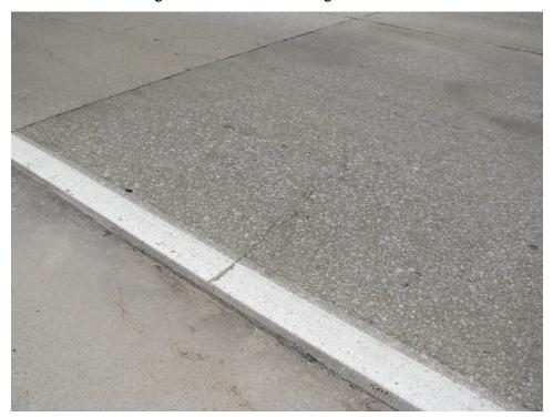
Figure 17.8 Corner cracking of UBCOA
