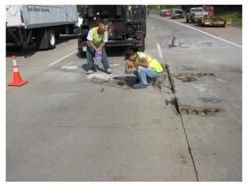
e. Delamination due to steel mesh located near the surface Andrew Bennett, Michigan DOT
