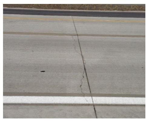
g. Joint spalling, possibly due to late sawing or saw cut not directly over existing pavement joint/crack Todd LaTorella, Missouri/Kansas Chapter, American Concrete Pavement Association
