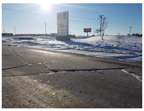
e. High severity cracking due to frost heave of the subgrade soil Michael Ayers, Global Pavement Consultants, Inc.
