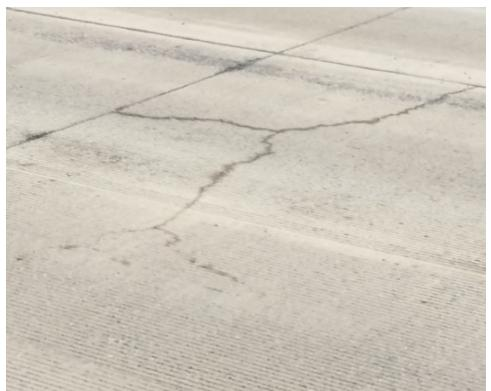
d. Multiple panel cracks near panel end due to debonding  $_{\rm Mark\ Snyder,\ PERC}$
