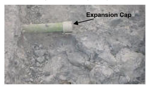
a. View of expansion cap on dowel bar Randy Riley, Illinois Chapter, Inc. – American Concrete Paving Association
