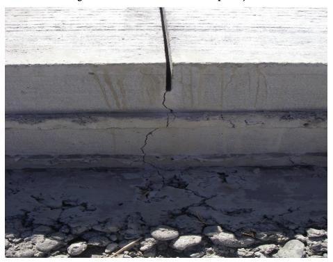
Figure 5.10 Saw cuts for weakened plane joint
