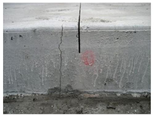
b. Slab cracking occurring parallel to weakened plane saw cut Derek Tompkins, American Engineering Testing, Inc.
