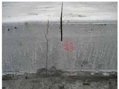
b. Slab cracking occurring parallel to weakened-plane saw cut, possibly due to late sawing or inadequate saw cut depth Derek Tompkins, American Engineering Testing, Inc.
