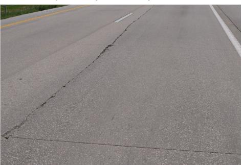
Figure 6.9 Longitudinal cracking in wheel line
