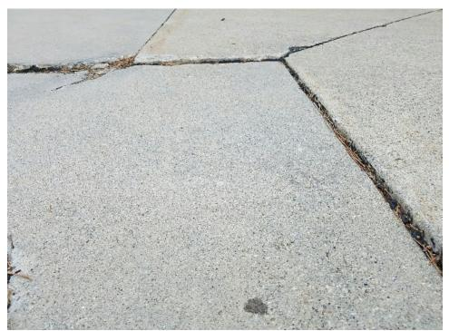
h. Settlement due to consolidation of the subgrade soil without significant traffic loading Dale Harrington, HCE Services
