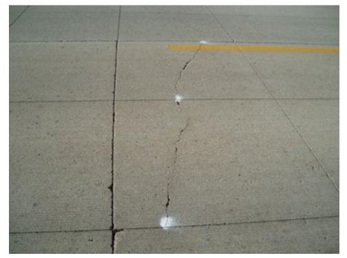
Figure 17.9 Mid-panel cracking due to inadequate support from the underlying HMA
