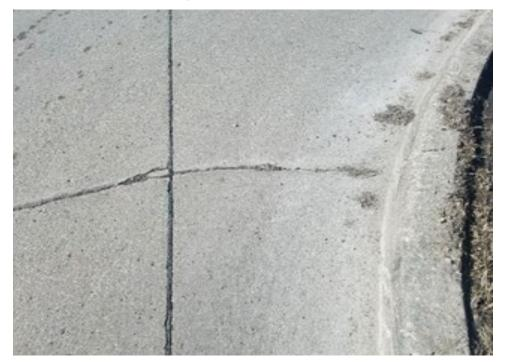
b. Cracking caused by lack of curb saw cut Dale Harrington, HCE Services
