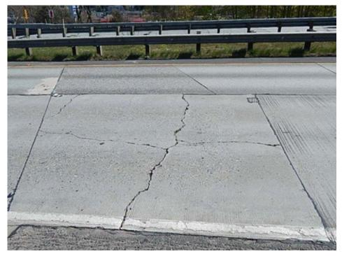
Figure 6.8 Shattered or broken panel
