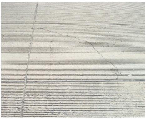
b. Corner crack in overlay due to debonding Mark Snyder, PERC
