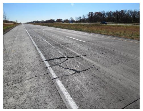
g. High severity cracking due to settlement and loss of support Tom Burnham, Minnesota DOT
