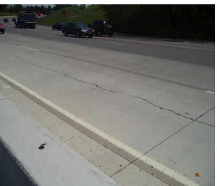
Figure 6.1 Longitudinal cracking in concrete pavements
