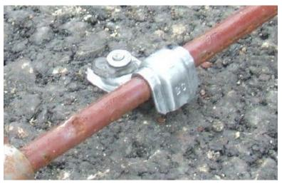
**b.** Anchor clip for dowel bar anchoring Eric Ferrebee, American Concrete Paving Association
