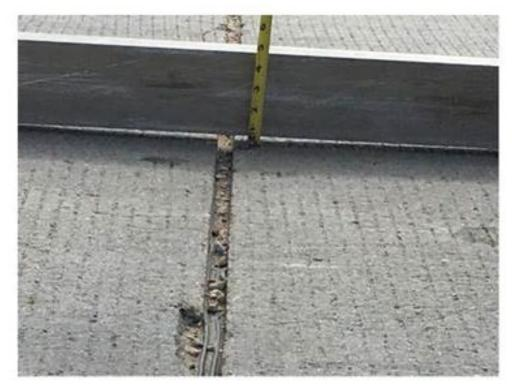
**b. Downward slab curvature visible at a transverse joint under straight edge** Todd LaTorella, Missouri/Kansas Chapter, American Concrete Pavement Association
