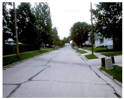
f. Reflective transverse and longitudinal cracking due to no placement of overlay joints Randy Riley, Illinois Chapter, Inc. – American Concrete Pavement Association
