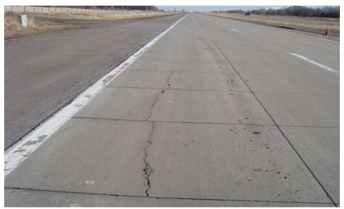
b. Longitudinal cracking in wheel path Kevin Merryman, Iowa DOT
