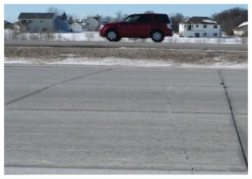
**f. Mid-panel cracking of UBCOC** Matt Zeller, Concrete Paving Association of Minnesota
