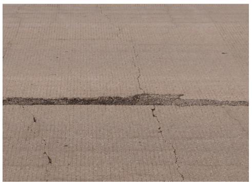
b. Moderate severity irregular transverse cracking in CRCP Global Pavement Consultants, Inc.
