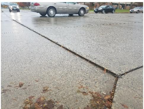
f. Settlement due to subgrade soil movement under traffic Dale Harrington, HCE Services
