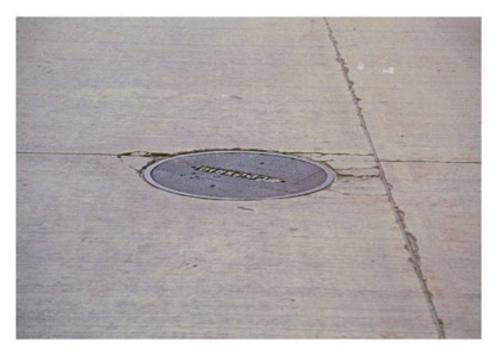
c. Cracking caused by lack of jointing to isolate a manhole ©2018 Applied Pavement Technology, Inc.
