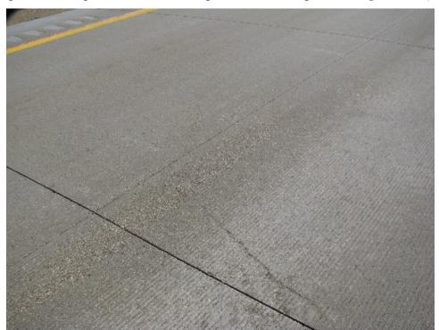
Figure 18.8 Irregular reflective cracking due to wrinkled geotextile separation layer
