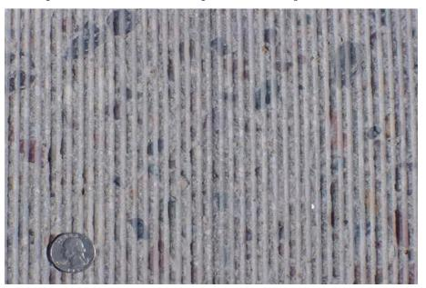
Figure 8.25 View of diamond ground concrete pavement surface
