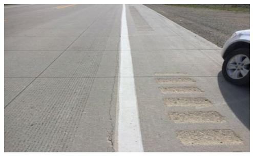
d. Longitudinal crack over widened section Kevin Merryman, Iowa DOT
