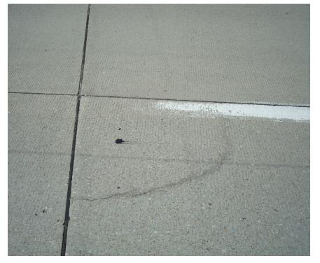
Figure 7.2 Corner cracks in concrete pavements
