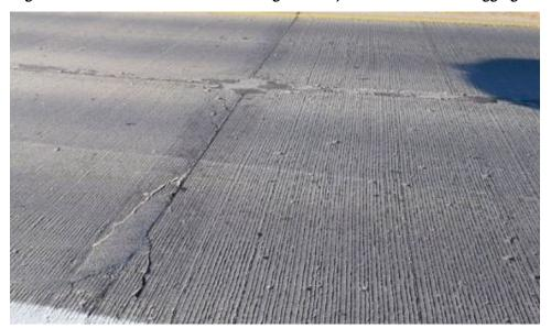
Figure 8.5 Saturated transverse and longitudinal joints with unsound aggregate
