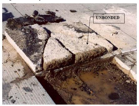
Figure 15.3 Examples of direct visual examination of bond interface
