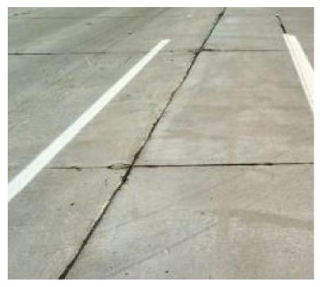
**f. Early saw joint raveling** National Concrete Pavement Technology Center
