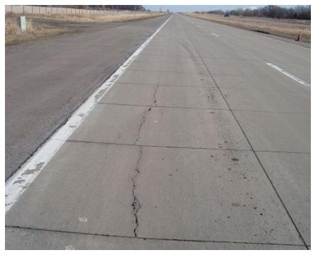
h. Longitudinal cracking in wheel path Julie Vandenbossche, University of Pittsburgh
