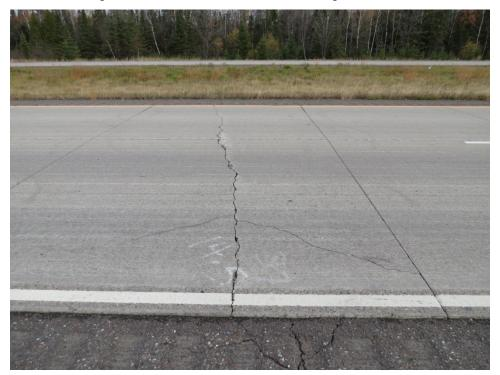
Figure 18.7 Transverse reflective cracking of UBCOC
