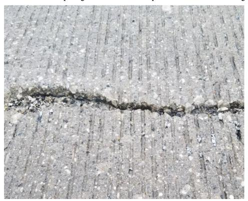
Figure 8.13 Deflection spalling of crack due to inadequate consolidation of the subgrade
