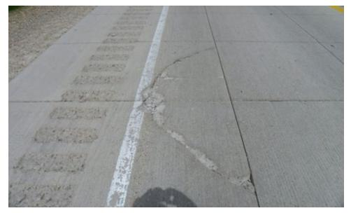
c. Diagonal longitudinal crack over widened section Kevin Merryman, Iowa DOT
