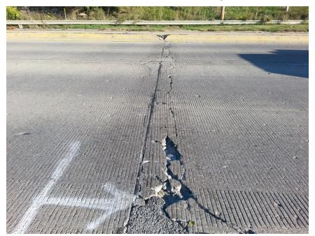
c. Saturated joint with unsound aggregate Snyder & Associates, Inc.
