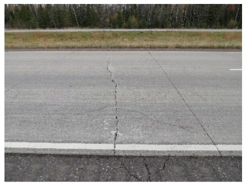
d. Transverse reflective cracking of UBCOC Tom Burnham, Minnesota DOT
