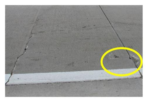
g. Transverse cracking of UBCOC due to severely misaligned dowels, yellow oval shows the exposed end of a misaligned dowel Andy Bennett, Michigan DOT
