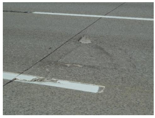
f. Typical pattern of delamination prior to surface loss  $$_{\rm Tom\ Yu,\ FHWA}$$
