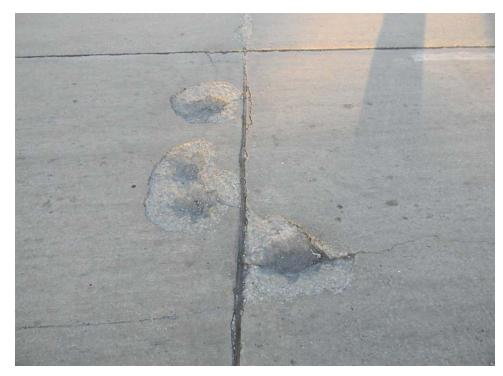
b. View of an improper placement of an expansion cap on the end of a dowel bar resulting in expansive pressure on the concrete causing spalling Randy Riley, Illinois Chapter, Inc. – American Concrete Paving Association
