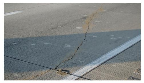
d. Longitudinal crack over dowels at JPCP transverse joint Mark B. Snyder, used with permission
