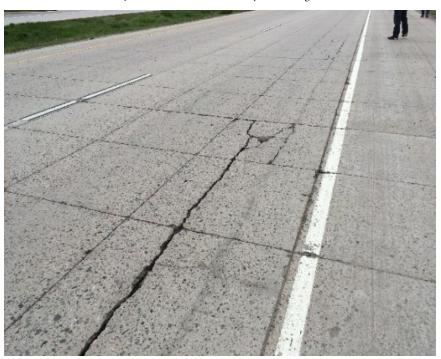
i. Multiple longitudinal cracking in wheel paths Mark Snyder, PERC
