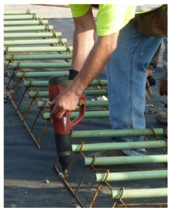
Figure 8.22 Typical dowel bar assembly with proper anchoring of the basket
