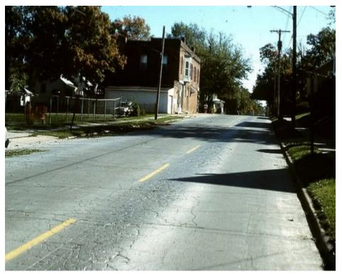
h. Longitudinal wheel path cracking due to debonding and fatigue cracking of overlay Randy Riley, Illinois Chapter, Inc. – American Concrete Pavement Association
