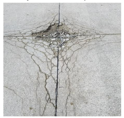
Figure 4.1 Various MRDs in concrete pavements
