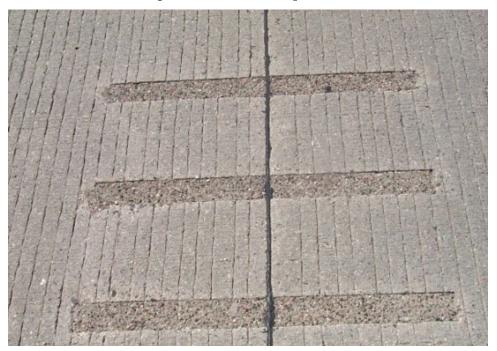
Figure 9.12 Cut slots in pavement
