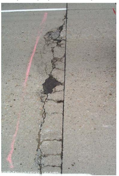
Figure 8.17 Spalling from dowel bar misalignment
