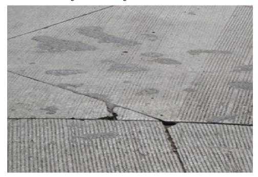
Figure 5.6 Cracking at urban intersections
