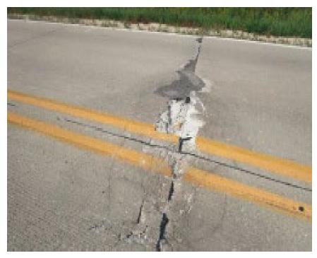
1. Compression at transverse joint due to slab expansion and adjacent joints not opening Matt Zeller, Concrete Paving Association of Minnesota
