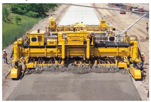
Figure 13.6 Vibration to fluidize and consolidate concrete
