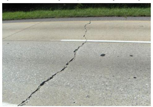
Figure 5.5 Transverse cracking caused by excessive slab lengths (20-foot panel)
