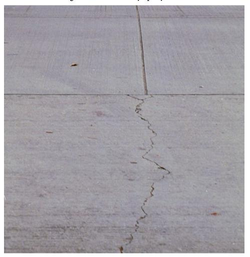
Figure 5.12 Transverse sympathy cracks
