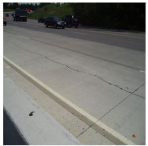
Longitudinal cracking is nearly parallel to the pavement centerline or lane-shoulder joint. Longitudinal cracks from surface cracks are covered in Chapter 2 and not in this longitudinal cracking chapter. This chapter covers full-depth cracks because they extend through the entire depth of the pavement. Other types of cracking include transverse, diagonal, and slab cracking—all of which are discussed in Chapter 5.
