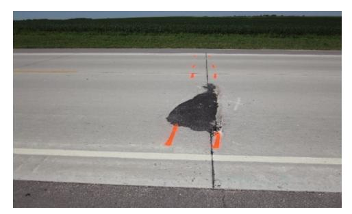
g. Transverse cracking due to severely misaligned dowels; paint marks show the dowel basket as located using GPR
