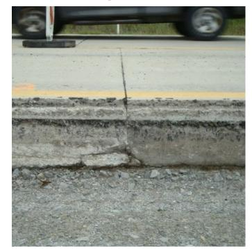
Figure 16.4 Bonded concrete overlay joint placed directly over full-depth repair joint in original pavement
