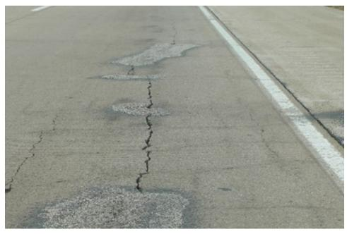
c. High severity longitudinal cracking in CRCP Global Pavement Consultants, Inc.
