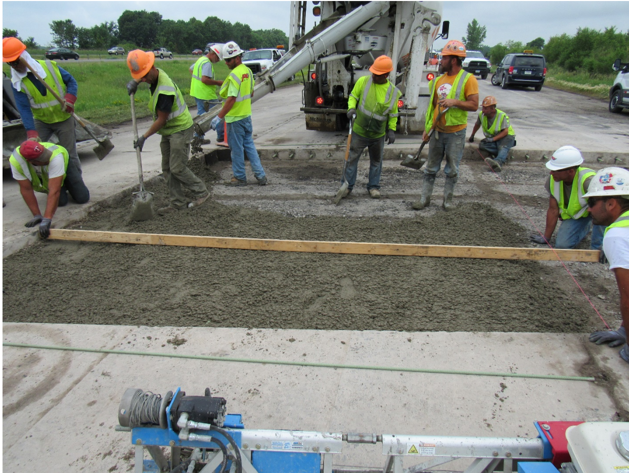
1 and 2 lift RCC (with dowel bars)
