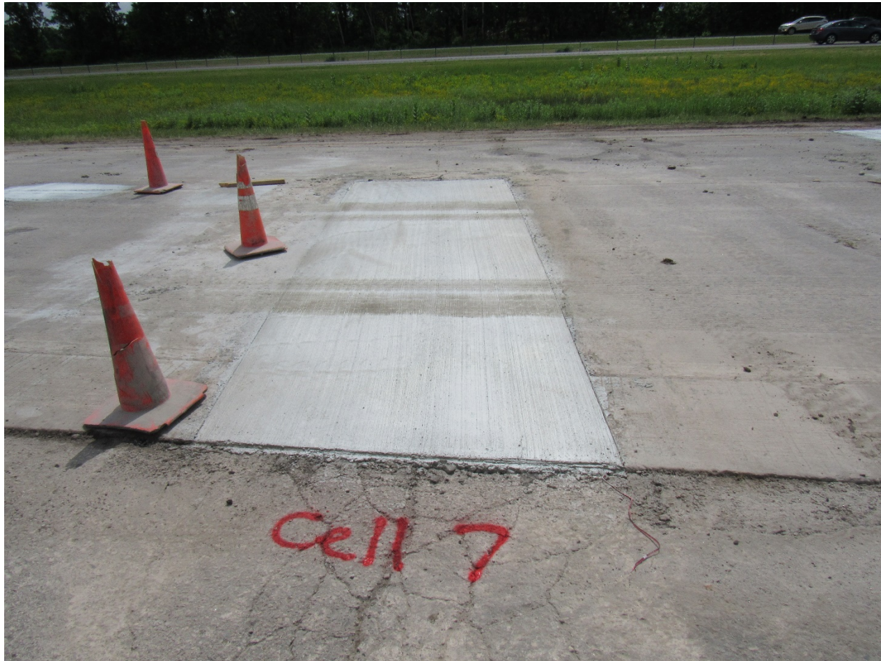
Full Depth Repairs
