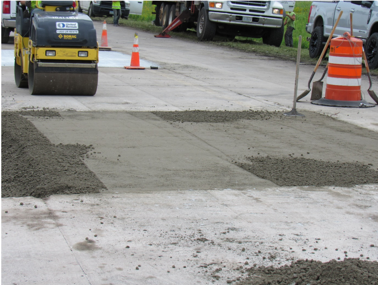
Small roller compaction
