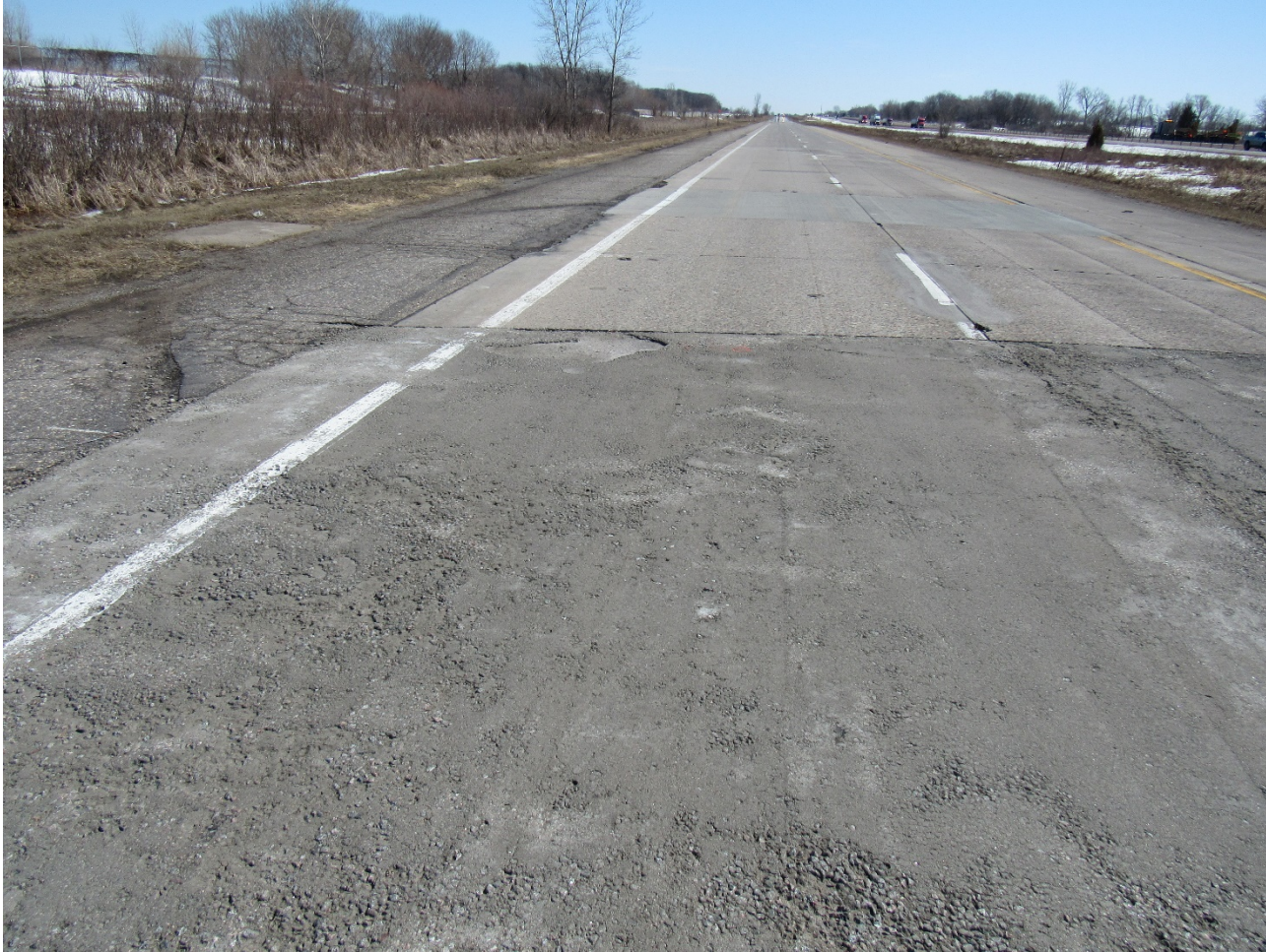
RCC repair condition - March 2019
