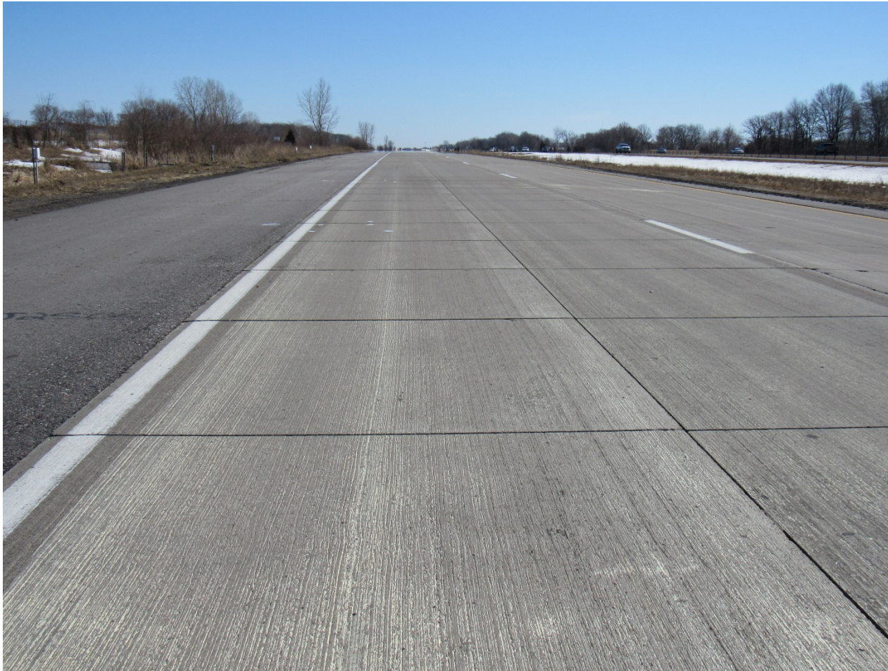
March 2019 condition: Faulted joints
