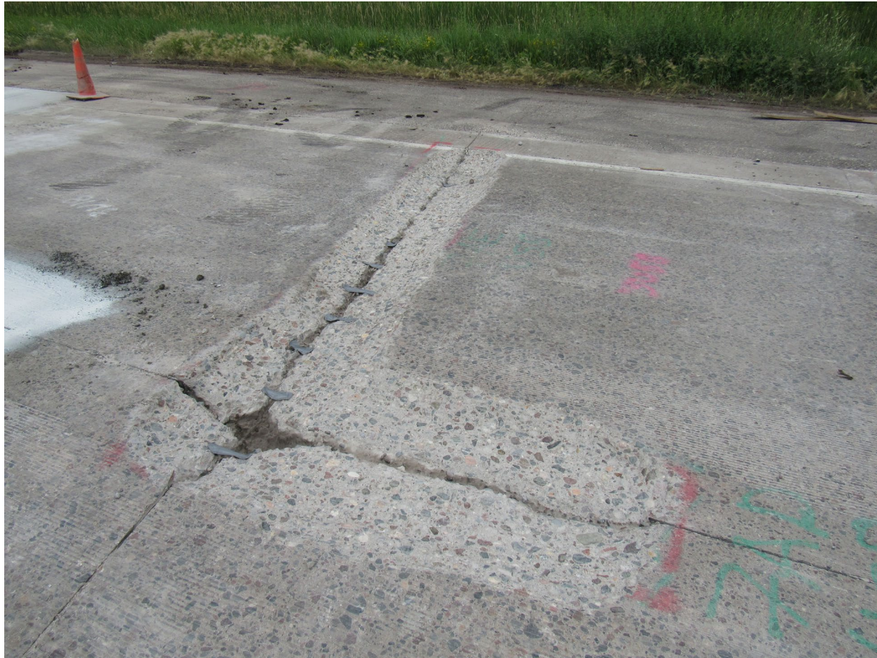
Partial Depth Repairs
