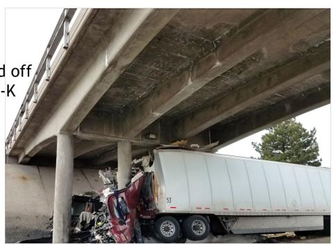
The force of the impact was so great that 2 of the 4 supports failed and collapsed.
