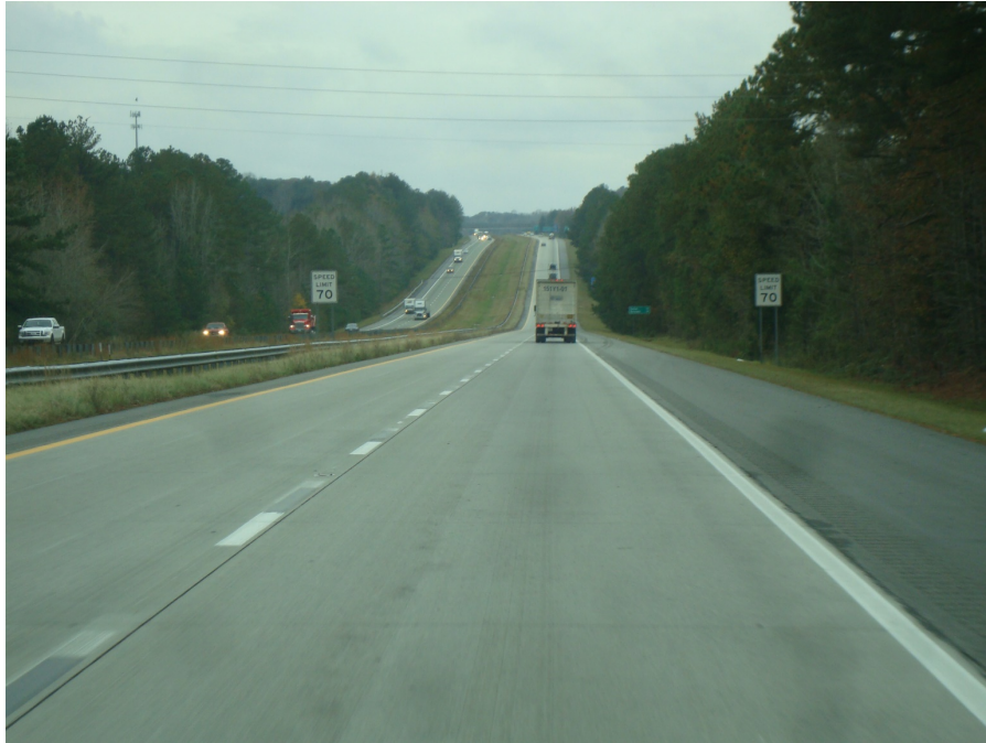
I-85, Granville Co., NC (Unbonded Overlay of CRCP CRCP Const. 1971 UBOL Const. 1997, DG 2010, Minor CPR 2015)
