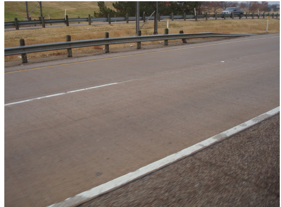
US 281 Wichita Falls, TX 2002 Bonded CRC Overlay of CRCP
