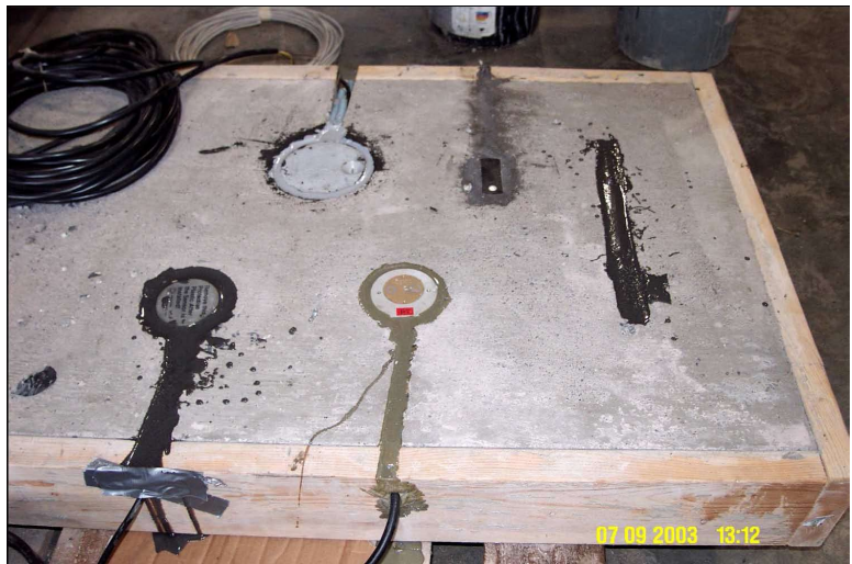
Concrete sensor installation
