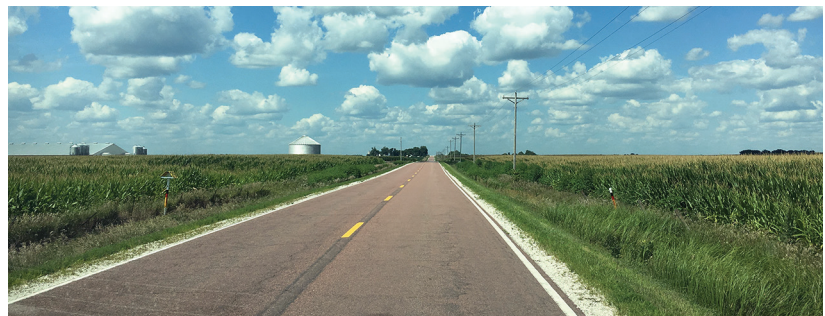
Micro-surfaced pavement in Hamilton County, Iowa
