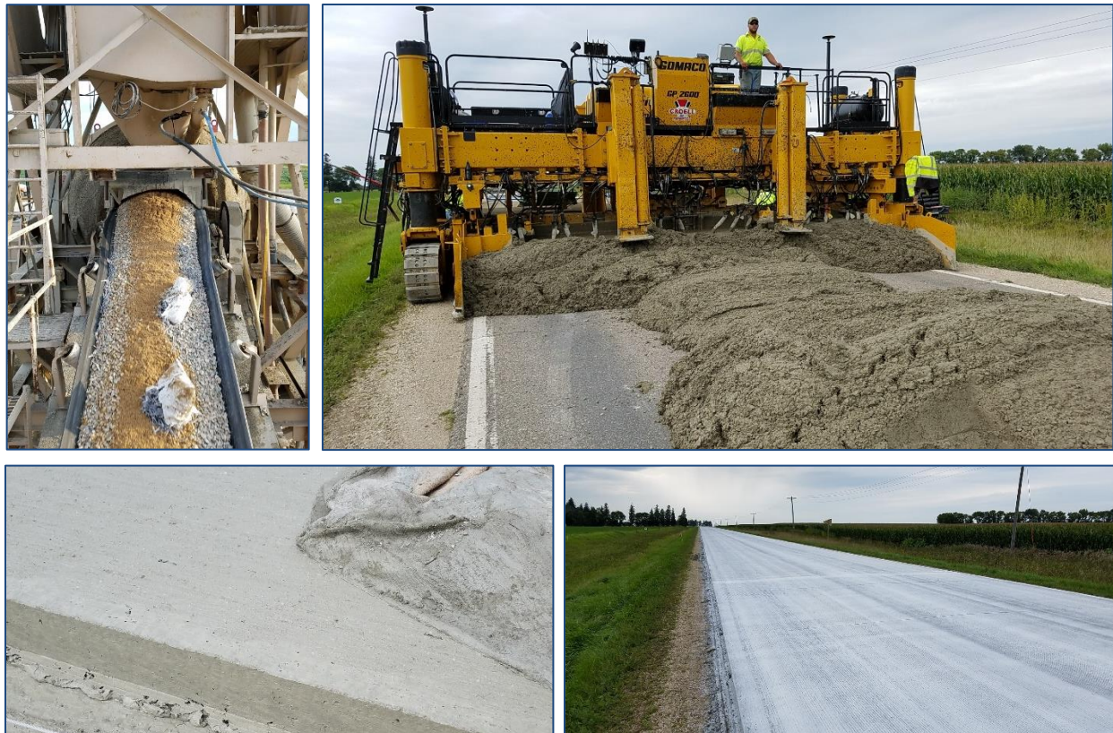
Figure 29. Mitchell County construction showing addition of fibers at the batch plant (top left), paving (top right), finishing with burlap drag (bottom left), and curing and tining (bottom right)
