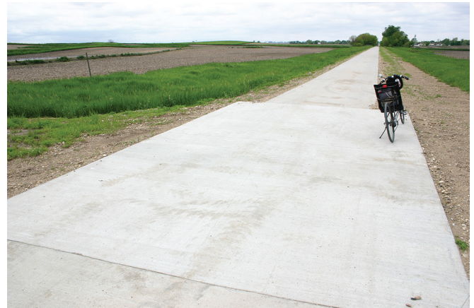
Figure 18. Thickened/widened section on field entrance crossings
