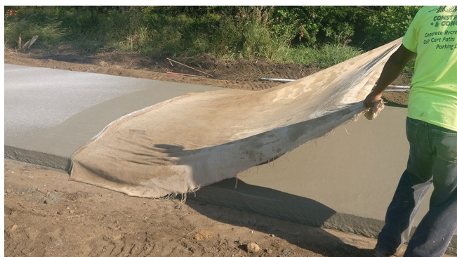
Figure 32. Manual burlap drag finish
