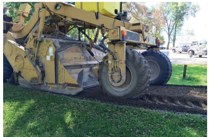
Brian Madsen, Howrey Construction
