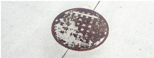
Figure 40. Utility access casting—completely within trail pavement slab
