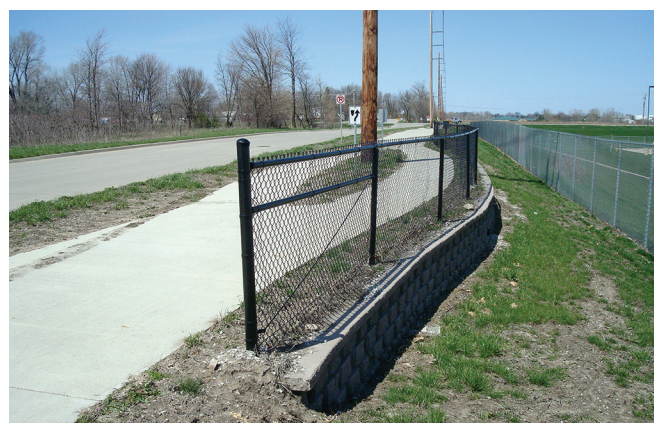
Figure 16. Barrier along the trail installed for safety
