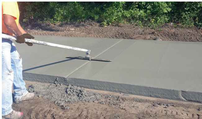
Figure 37. Hand-tooled joints prior to saw operations
