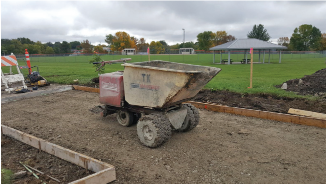
Figure 27. Buggies provide efficient concrete delivery
