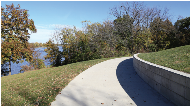
Figure 25. Combined retaining wall and trail
