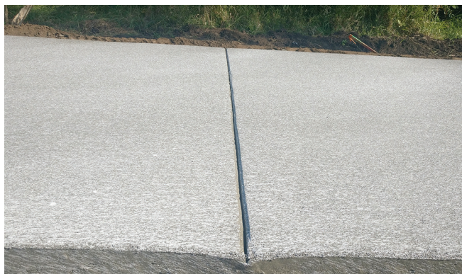
Figure 38. Tooled transverse joint in fresh concrete
