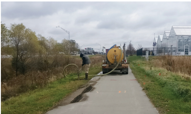
Figure 11. Utility potholing
