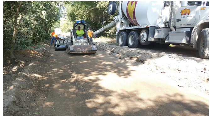
Figure 26. Concrete trail construction
