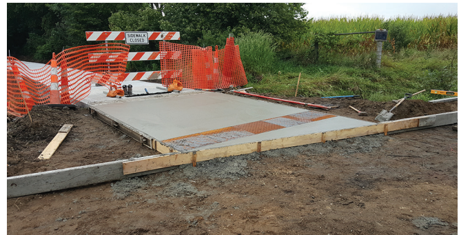
Figure 43. ADA ramp in rural section
