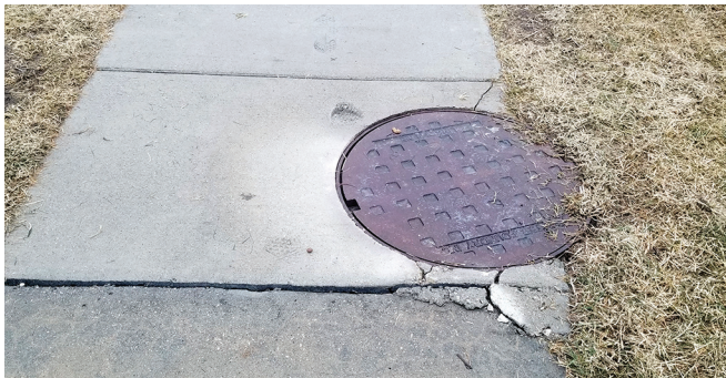
Figure 41. Utility access casting—partially within trail pavement slab
