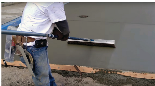
GBR Paving ( https://www.youtube.com/watch?v=Nr24a2wgdBY )
