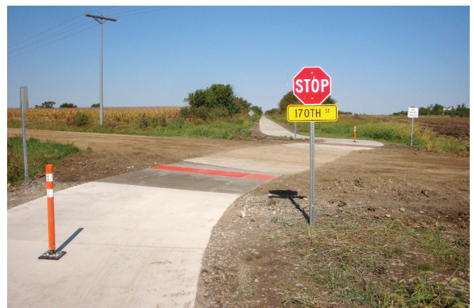
Figure 19. Sign and bollard installed at intersection/crossing
