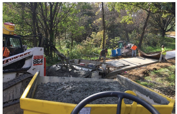
Brian Madsen, Howrey Construction
