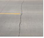
ing is oriented obliquely across a slab, at roughly a 30–60 degree angle from the pavement centerline. Slab cracking may also develop longitudinally, in which the crack is oriented parallel to the pavement centerline. This chapter focuses on transverse and diagonal cracking, with Chapter 6 providing detailed information on longitudinal cracking.
