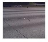
sides are rarely less than 1 ft (0.3 m) and are always less than one-half the width of the slab (by definition) on each side of the corner. Cracks with longer legs are considered diagonal cracks (see Chapter 5).
