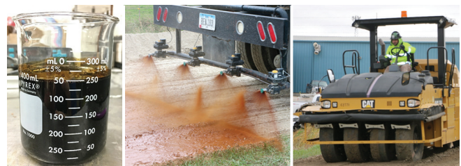
Lignosulfonate test section construction
