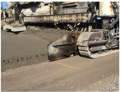
The Transtec Group, Inc. Figure 13. Properly graded and stable paver track line
