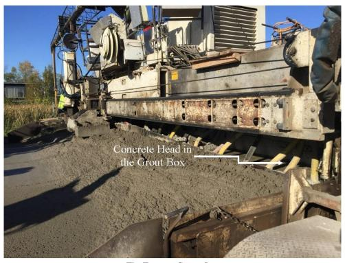
The Transtec Group, Inc. Figure 12. Maintaining the concrete head in the grout box
