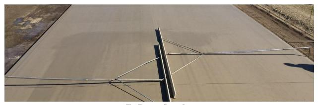
The Transtec Group, Inc. Figure 23. Hand finishing with two 16 ft straightedges
