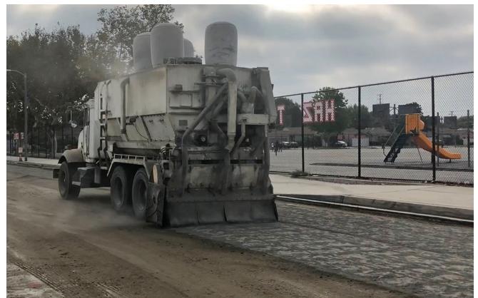
© 2020 Pavement Recycling Systems (PRS) Inc., used with permission
