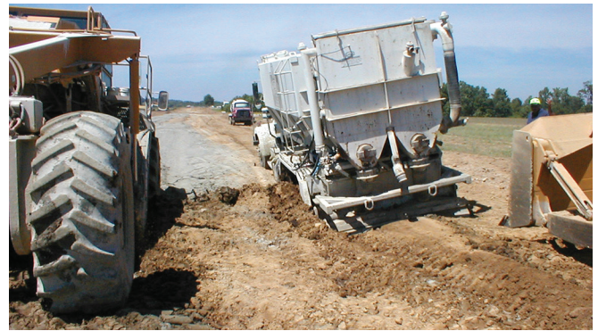
Figure 6.5. Weak materials evidenced during modification
