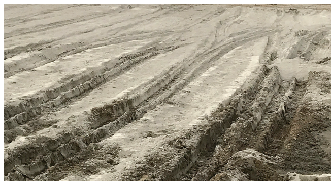
Figure 6.7. Subgrade after cement application
