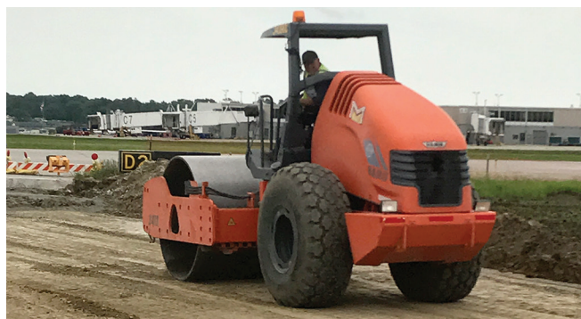
Figure 6.9. Compacting cement-stabilized subgrade
