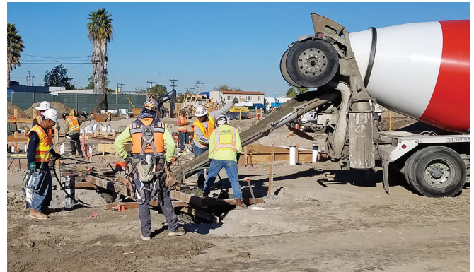
© 2020 Pavement Recycling Systems (PRS) Inc., used with permission
