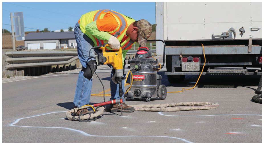
Typical corrective maintenance for damaged concrete: epoxy injection
