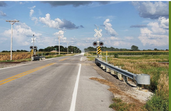
Longitudinal guardrail protecting a signal mast in Elkhart, Iowa
