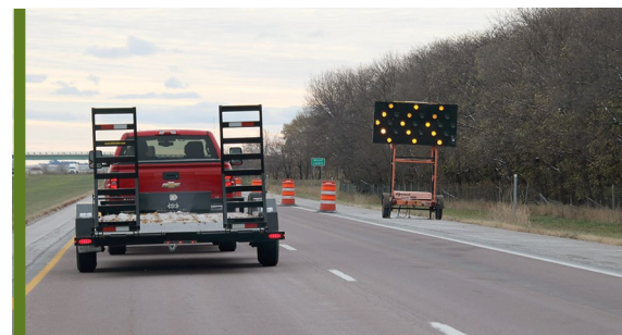
Smart arrow board at the beginning of a work zone in Iowa Project: Developing a Research-Grade Iowa Work Zone Database Sponsor: Iowa DOT
