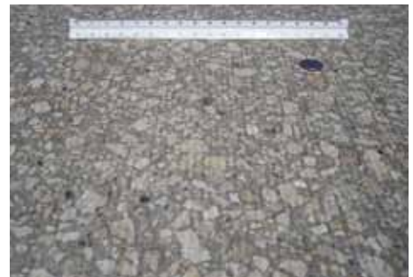
Figure 6. CPSCP Section 205-E having small within-section variability with OBSI level versus distance (left) and photo of the pavement surface texture (diamond ground) (right)
