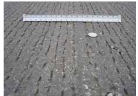
Figure 7. CPSCP Section 205-K having large within-section variability with OBSI level versus distance (left) and photo of the pavement surface texture (longitudinally-tined) (right)
