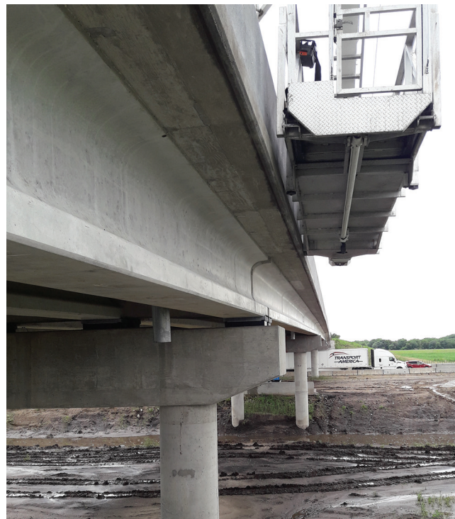
Gauge installation for live load testing on the new County Road E-57 bridge over I-35 in 2017
