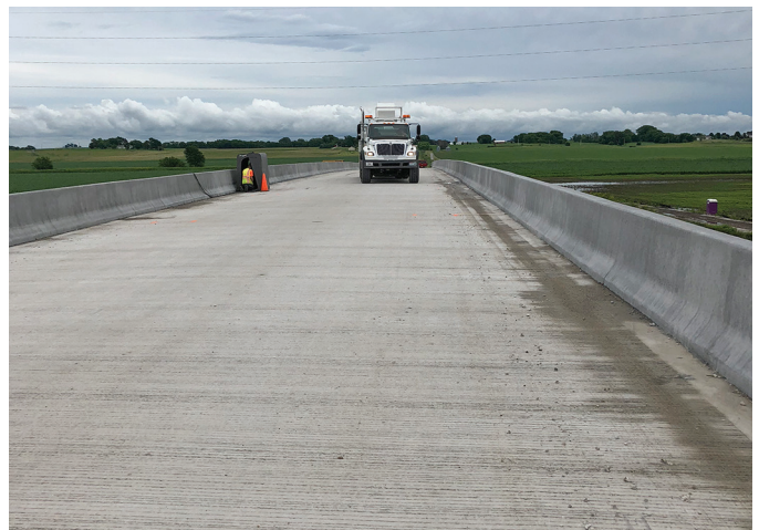
Live load testing the County Road E-57 bridge over I-35
