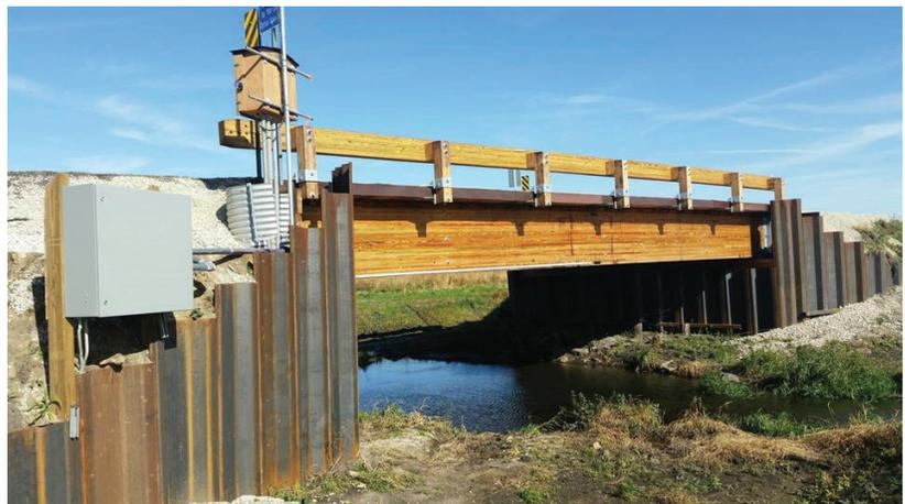
*The Buchanan County Catt Bridge is a geosynthetic-reinforced soil-timber bridge on 215th Street, east of Independence, Iowa*
