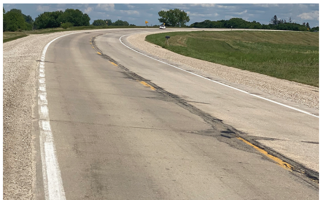
Greg Mulder, Iowa Concrete Paving Association, used with permission
