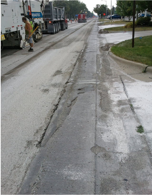
Figure 8.15. Results of a typical concrete pavement milling operation
