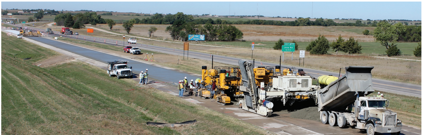
Figure C.8. Placement of a thin COC-B overlay
