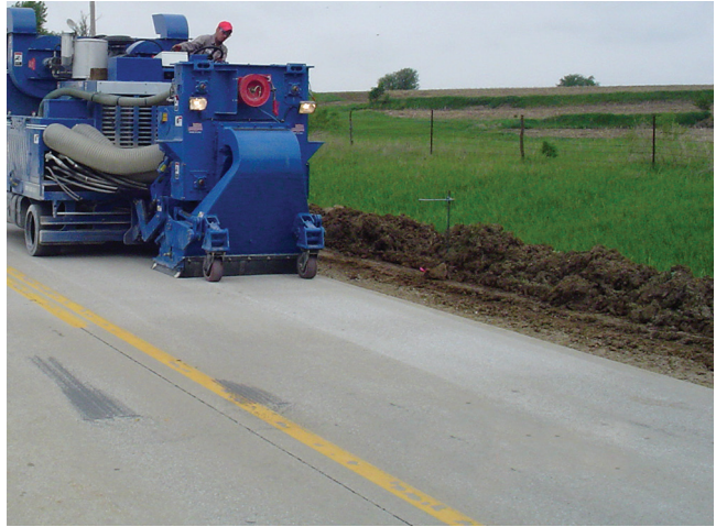
Figure C.6. Shotblasting of a concrete surface
