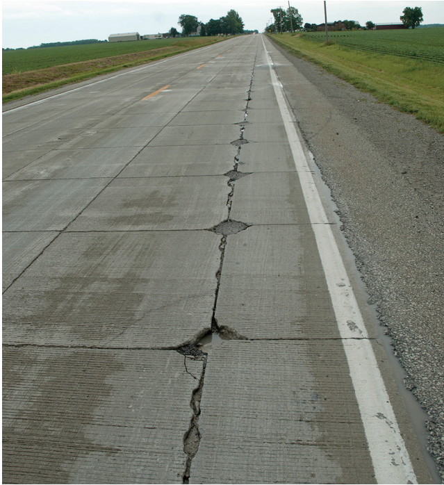
Figure 3.2. Concrete overlay on composite pavement photographed in 2012 after 13 years in service, with the overlay exhibiting interior corner deterioration due to longitudinal joints in the wheel paths
