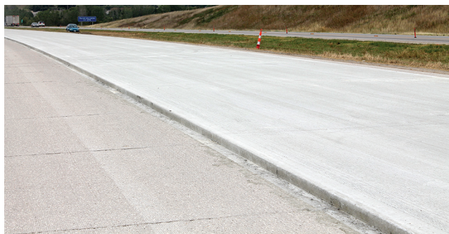
Figure C.1. Thin bonded overlay of structurally sound concrete pavement
