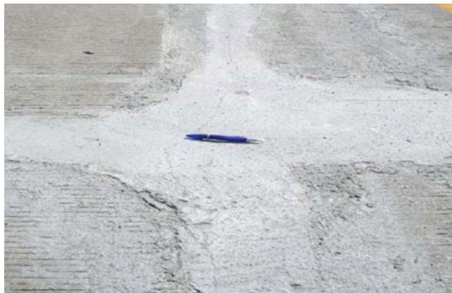
Figure 8.5. Deteriorated joints in existing concrete pavement cleaned and filled with flowable mortar
