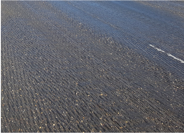
Figure 8.3. Asphalt surface milled to enhance bonding with a concrete overlay
