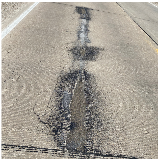
Figure C.2. Deteriorated longitudinal crack in a COC–B overlay
