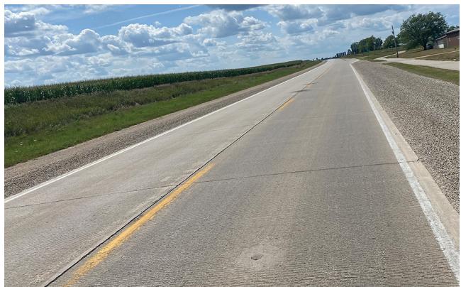
Greg Mulder, Iowa Concrete Paving Association, used with permission
