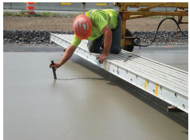
Figure 8.10. Manual verification of dowel placement
