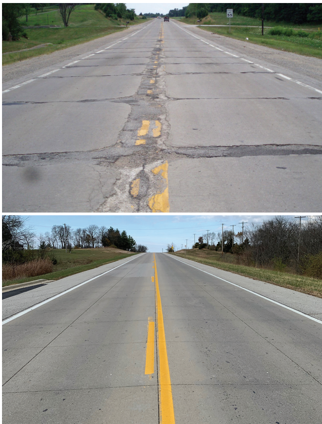
Figure 5.3. Route D existing concrete in deteriorated condition in 2007 (top); 5 in. unbonded overlay constructed on Route D in 2008 (bottom, photo taken in 2020)
