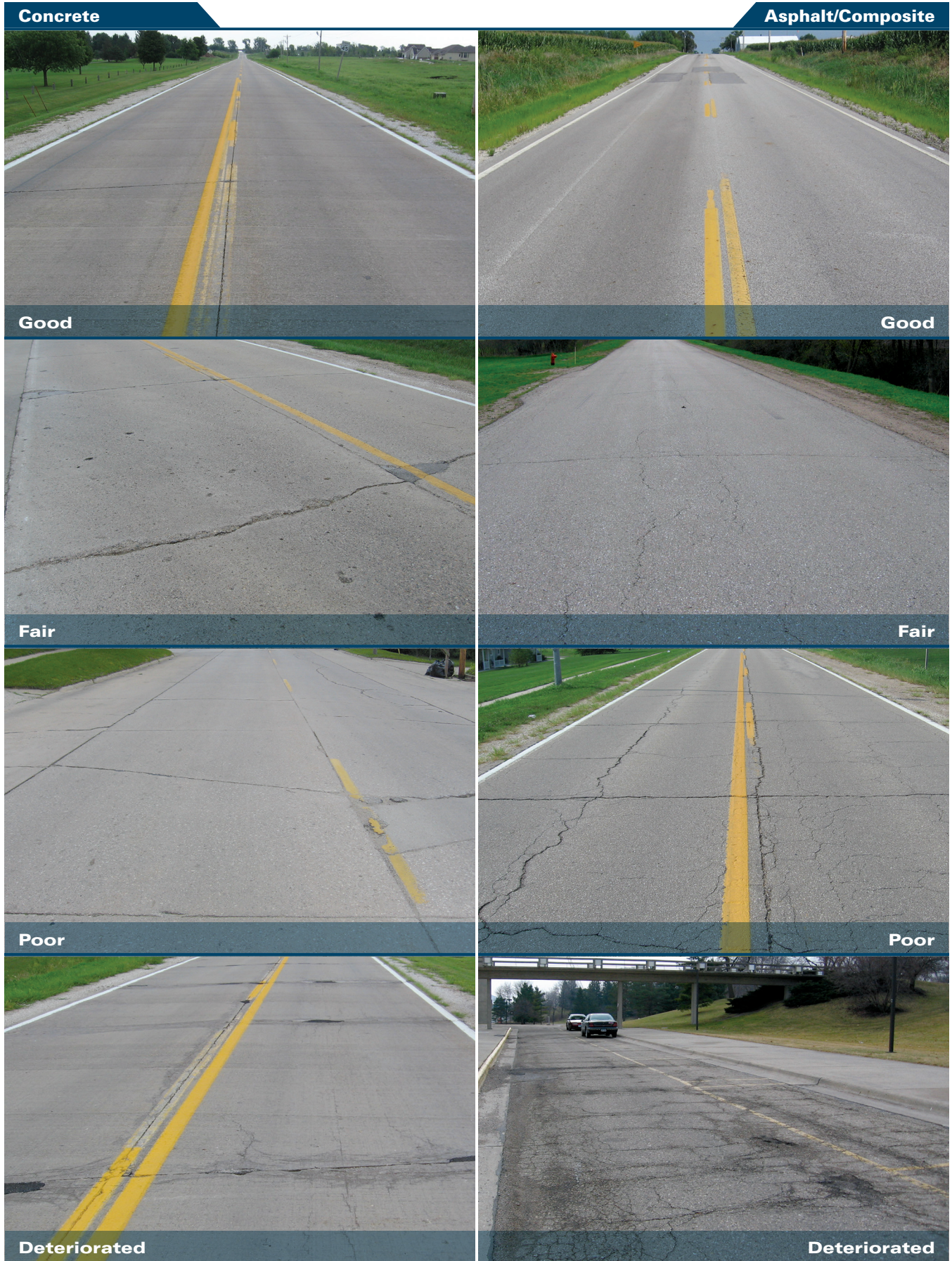
Figure 2.1. Examples of determining existing pavement type and condition
