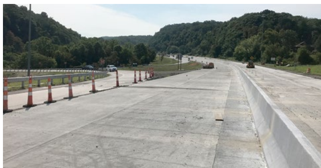
Figure 51. Completed COC-U overlay on US 30, with ramp movements maintained during construction
