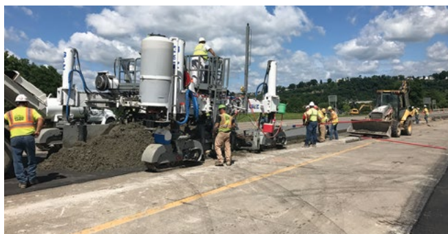
Figure 50. COC-U overlay placement on US 30
