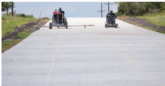
Figure 54. Sawing operations on SH51 timed to prevent random cracking
