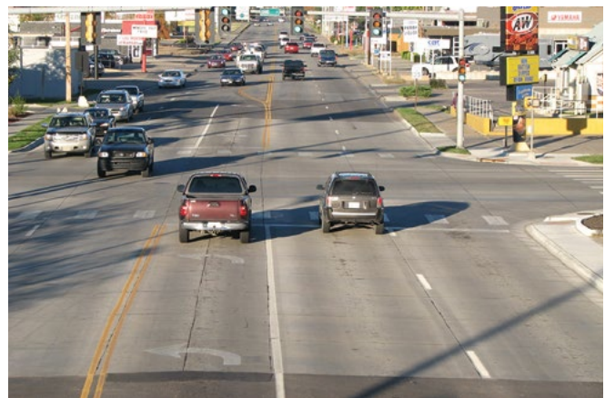
Figure 43. Finished project at the intersection of E. Crawford Street and S. Ohio Street, including new curb and gutter sections, inlets, and sidewalks
