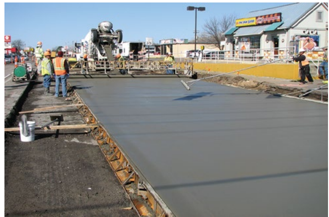
Figure 42. Fixed-form construction of the COA-U overlay at the intersection of E. Crawford Street and S. Ohio Street
