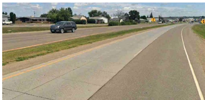
Figure 39. COA–B overlay placed in the left lane of the West Dakota Parkway just west of a major left-turn movement, with the existing inside shoulder and less traveled right lane and shoulder undisturbed during overlay construction
