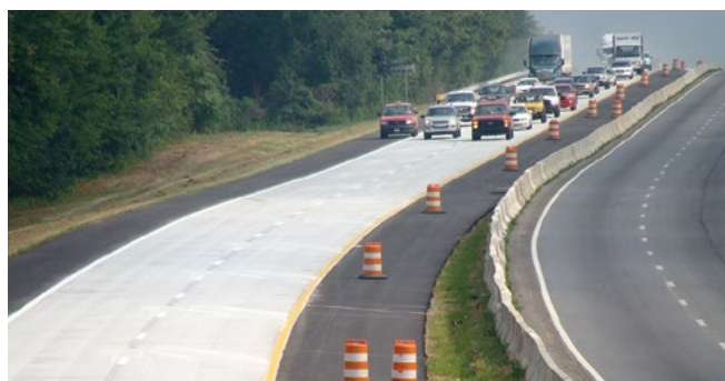
Figure 21. Southbound lanes of I-77 opened to traffic, showing a median detour that had been carrying southbound traffic during COC-U overlay construction
