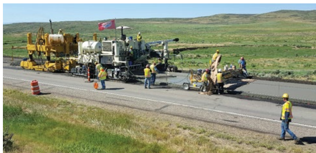
ACPA, used with permission (Castle Rock Construction Company)
