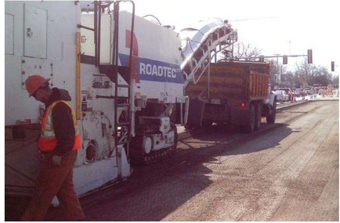
Figure 41. Milling of the existing asphalt overlay(s) at the intersection of E. Crawford Street and S. Ohio Street
