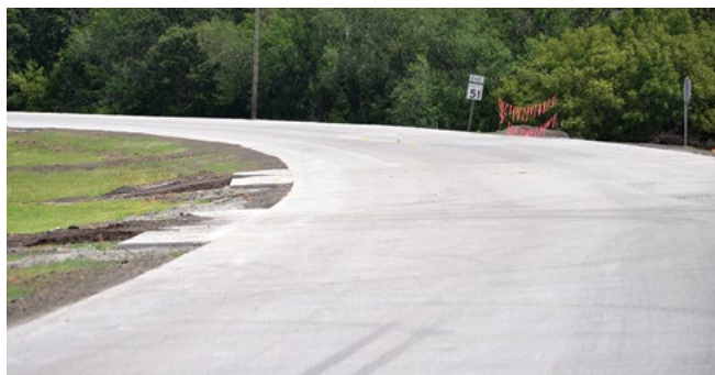
Figure 55. Completed COA-B overlay on SH51, with drainage structures extended to accommodate widening of the existing roadway
