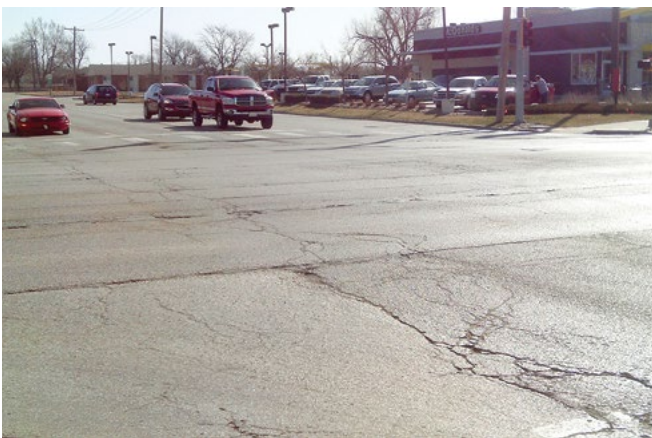
Figure 40. Pavement condition at the intersection of E. Crawford Street and S. Ohio Street prior to the overlay
