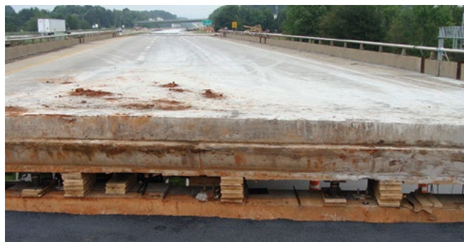
Figure 20. Bridge jacking to match the new COC-U overlay elevation on I-77
