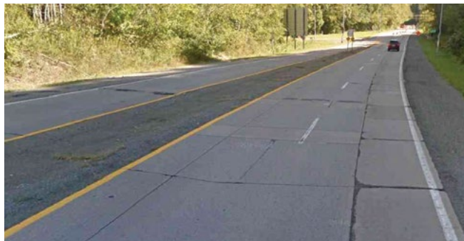
Figure 48. Existing pavement condition on US 30 prior to overlay placement (September 2016)
