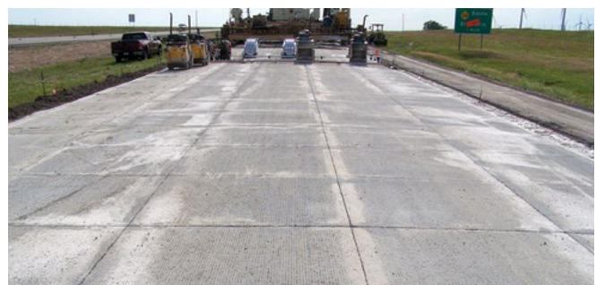
Figure 25. Longitudinal and transverse joint sawing caught up to the paving operation on I-70, with eight saws required to keep pace
