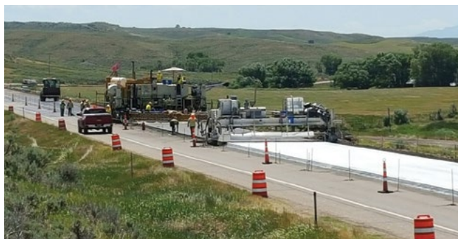
ACPA, used with permission (Castle Rock Construction Company)
