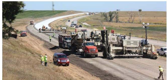
Figure 23. COA–B overlay construction on I-70, with traffic using a contraflow pattern
