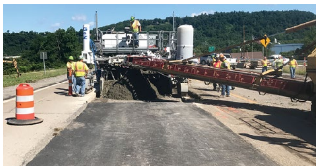
Figure 49. Paving of the COC-U overlay on US 30 over an asphalt separation layer
