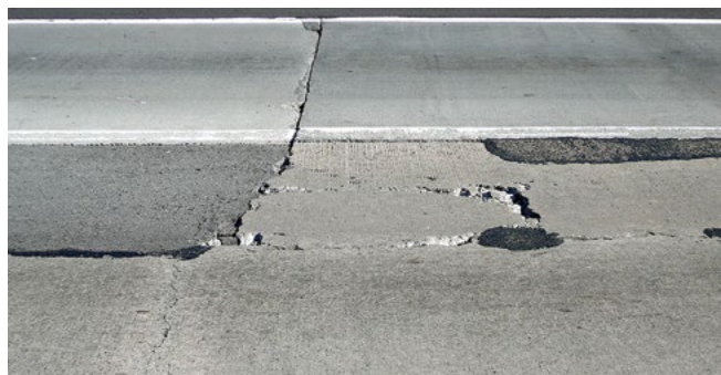
Figure 18. Existing pavement condition on I-77, with punchouts, ruptured steel, and faulting at cracks
