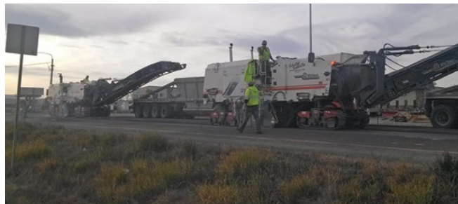
Figure 36. Milling of the West Dakota Parkway
