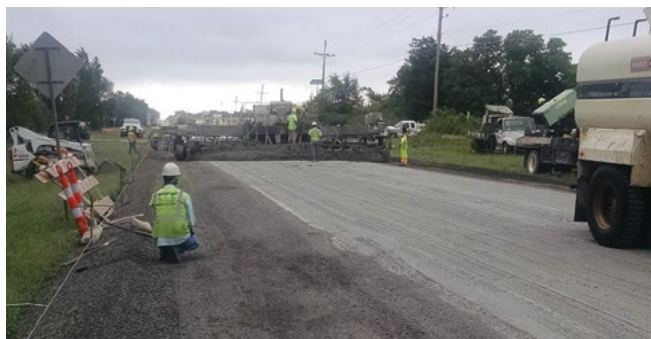
Figure 52. Full-width paving of the COA-B overlay on SH51, with the milled surface of the existing pavement visible
