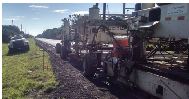
Figure 53. COA-B overlay placement on SH51, with the texture and curing operations following closely behind the paving
