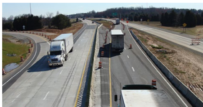
Figure 19. COC-U overlay construction on I-77 with two-lane crossover
