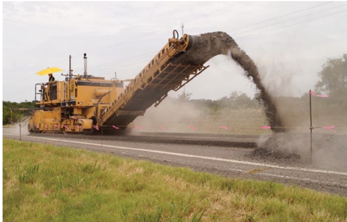
Brent Burwell, ACPA, OK/AR Chapter, used with permission Figure 17. Profile milling of the existing asphalt pavement
