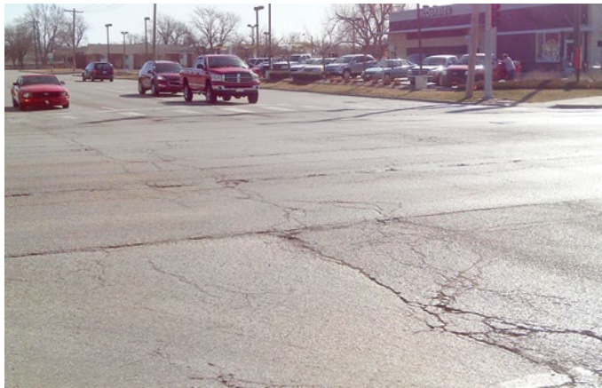
ACPA, used with permission (Pavers Inc.)
