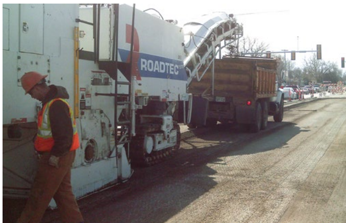
ACPA, used with permission (Pavers Inc.)
