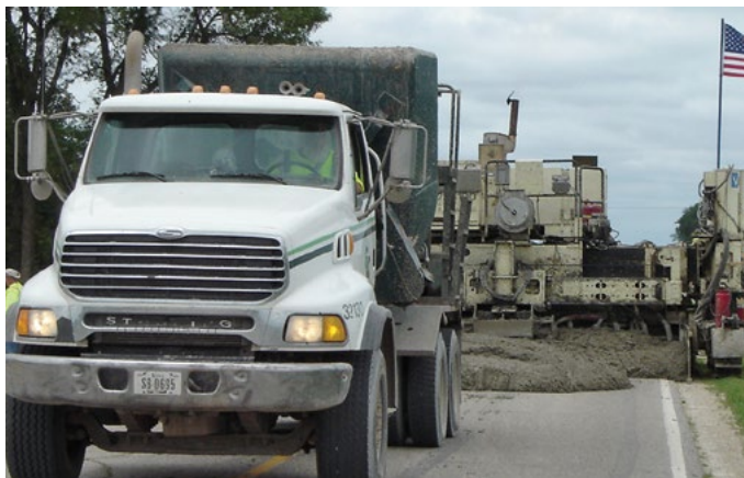
Figure 22. Paving of the unbonded concrete overlay on the existing roadway, which was not milled before paving
