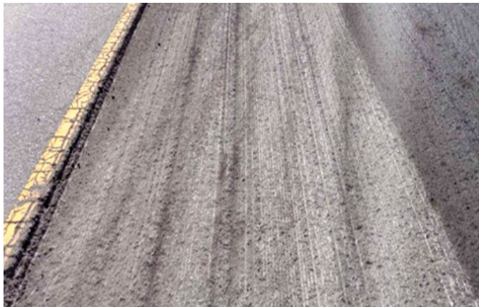
Castle Rock Construction, provided by Angela Folkestad, ACPA, CO/WY Chapter, used with permission
