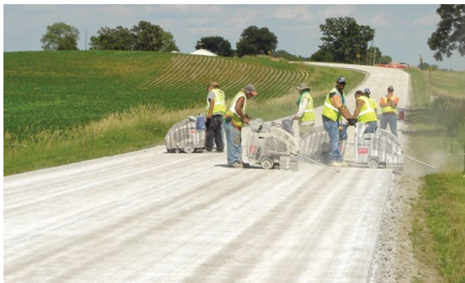
Figure 23. Transverse and longitudinal joints being sawed at a spacing of 6 ft center on center, with up to 54,000 lineal feet of joint sawing completed on high-production paving days
