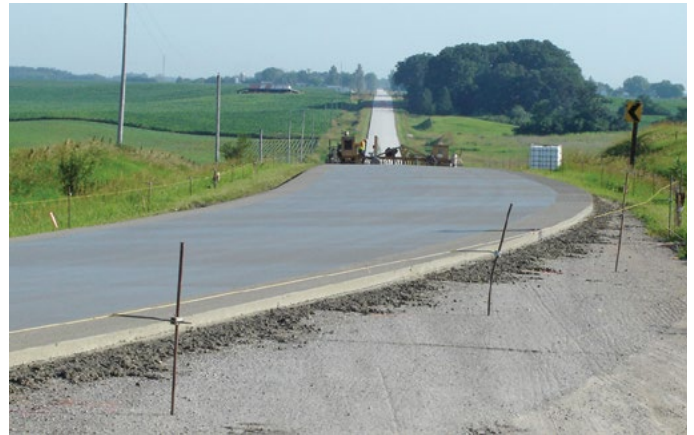
Figure 24. Variable-depth concrete used to upgrade curves from a normal cross slope to a super-elevated section
