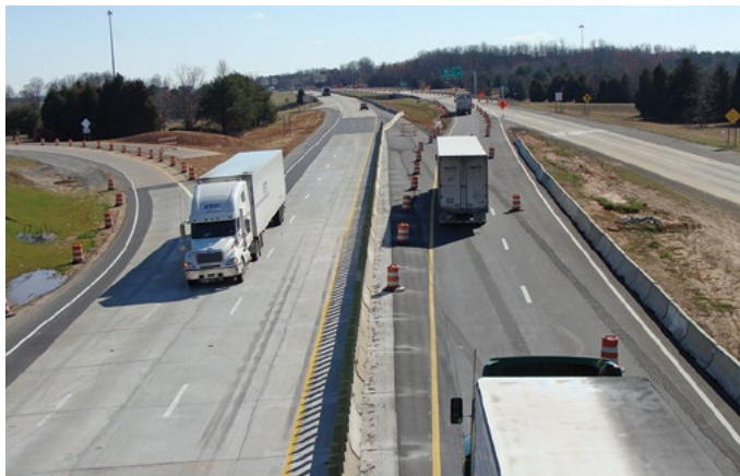
ACPA, used with permission (The Lane Construction Corporation)
