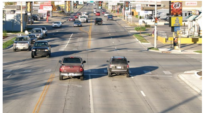
ACPA, used with permission (Pavers Inc.)
