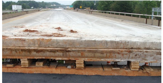
ACPA, used with permission (The Lane Construction Corporation)
