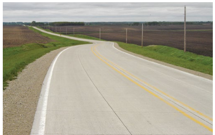
Figure 25. Finished concrete overlay approximately one year after construction
