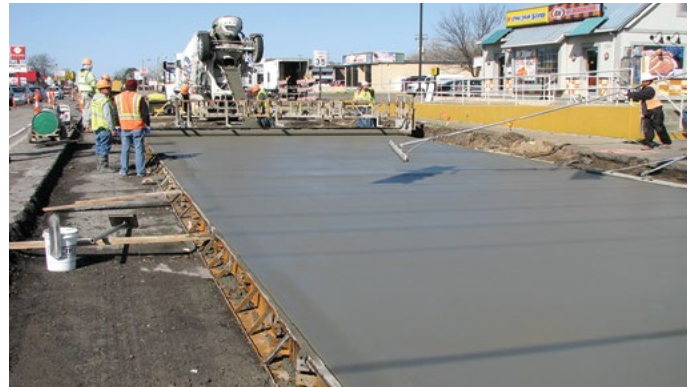
ACPA, used with permission (Pavers Inc.)
