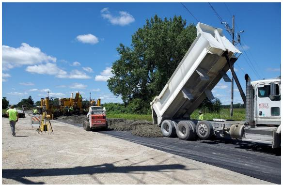
Image taken on July 22, 2020, Dan King, Iowa Concrete Paving Association Figure 11. Thin black geotextiles placed over existing ACC pavement
