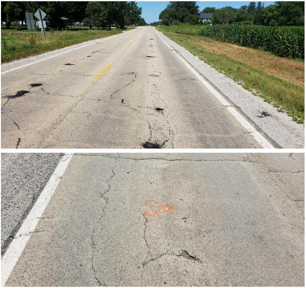
Images taken on July 10, 2020 Figure 9. Existing condition of CR D-16 with ACC surface
