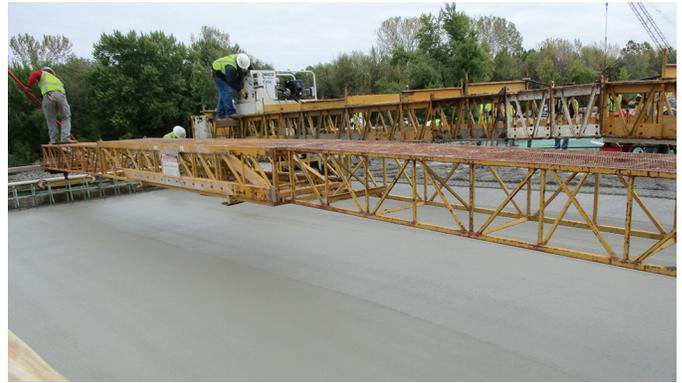
*Concrete deck placement in Iowa like that observed and studied for construction factors as part of this study*
