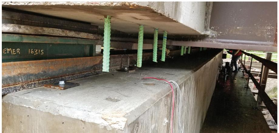
*Closure joint between super- and sub-structure during the construction of a multi-span bridge using SIBC on IA 1 over Old Man's Creek southwest of Iowa City*
