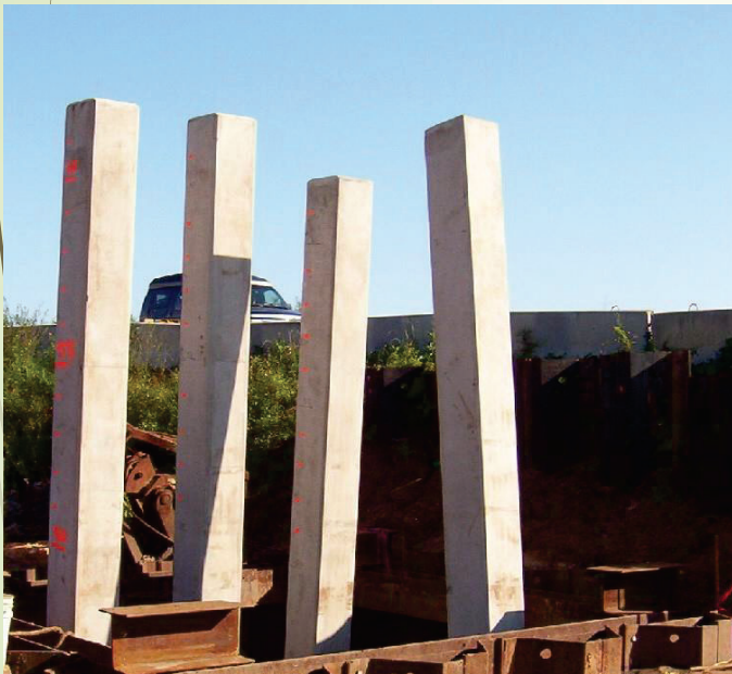
Fish River Bridge in Florida. Concrete has 12% metakaolin.
