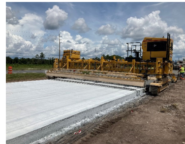
US Highway 301, Clay County, Florida
