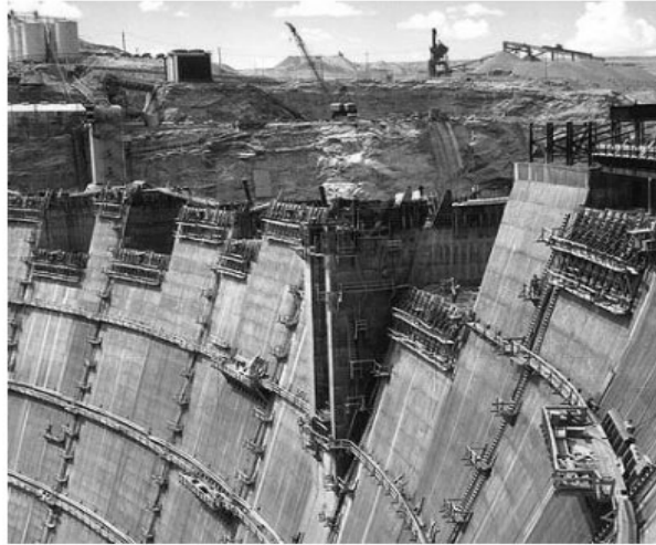
File photo: Construction of Glen Canyon Dam, Page, Arizona, circa 1960
