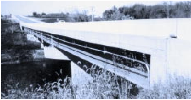
FIGURE 1 Boone River bridge on IA-17.
