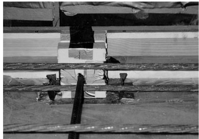
FIGURE 7 Shear-key and pocket forming.
