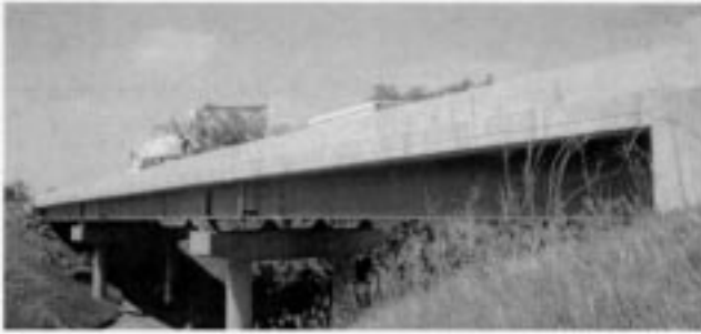
FIGURE 2 I-80 Bridge No. 7804.8L080.
