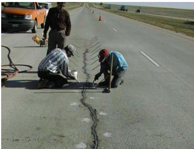
FIGURE 4. Installation of Stitches on I-70 at Agate
