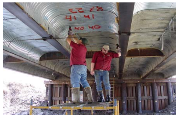
(b) Removing the arched formwork
