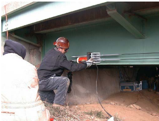
(c) Application of P-T force in West-end span
