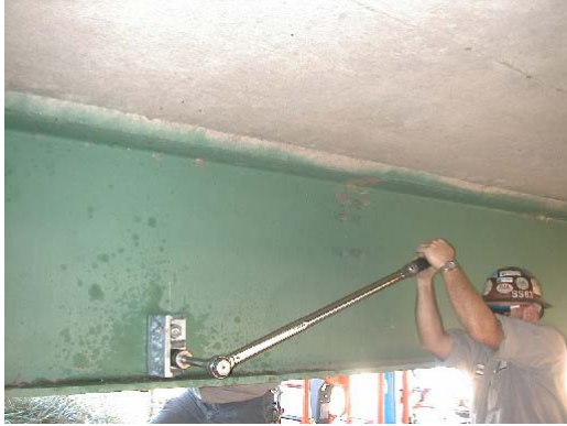
(a) Installation of anchorage assembly
