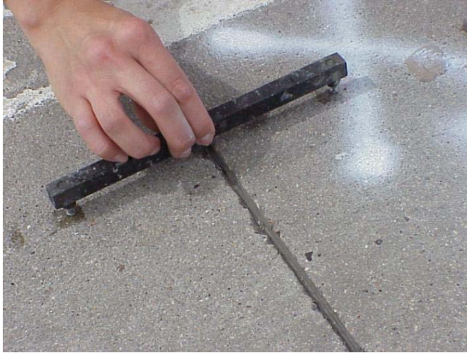
FIGURE 3. Reference Pins Installed Across a Joint
