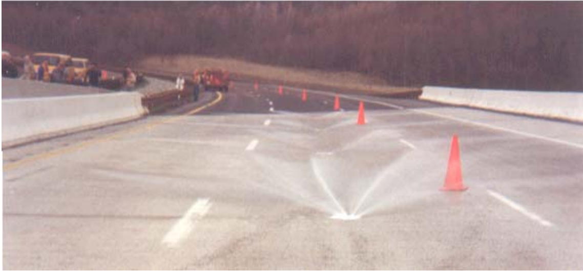
FIGURE 1. A Bridge-Deck Anti-Icing System in Operation (Source: Odin Systems International, Inc.)
