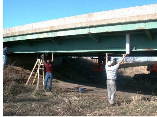
(b) Placement of CFRP rod
