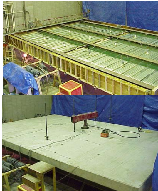
(a) Formwork and reinforcing before concrete placement
