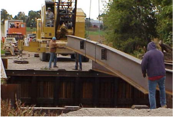
(a) Setting the girders into place
