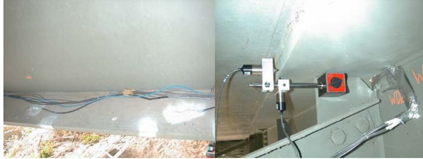
FIGURE 8. Photographs of Longitudinal Strain Gages and Out-Of-Plane Transducers
