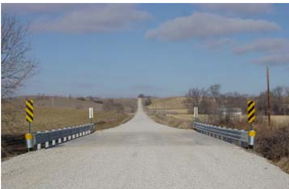
(a) Finished MBISB Demonstration Bridge
