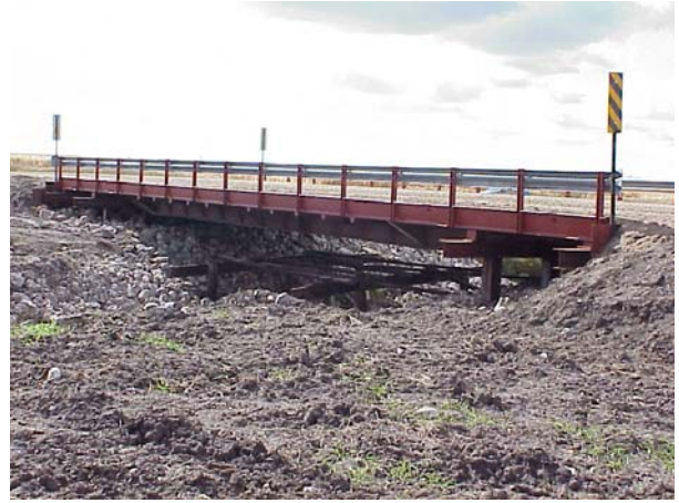
(b) Winnebago County Bridge
