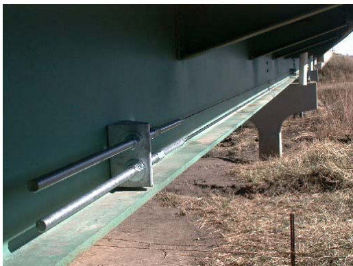
(a) CFRP Rods on West-end span
