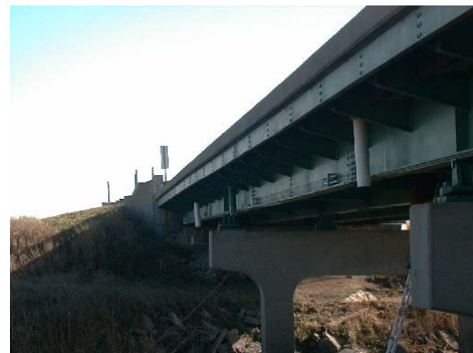
(b) CFRP rods on Center span
