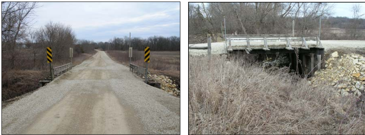
Figure 6. Existing bridge, Madison County
