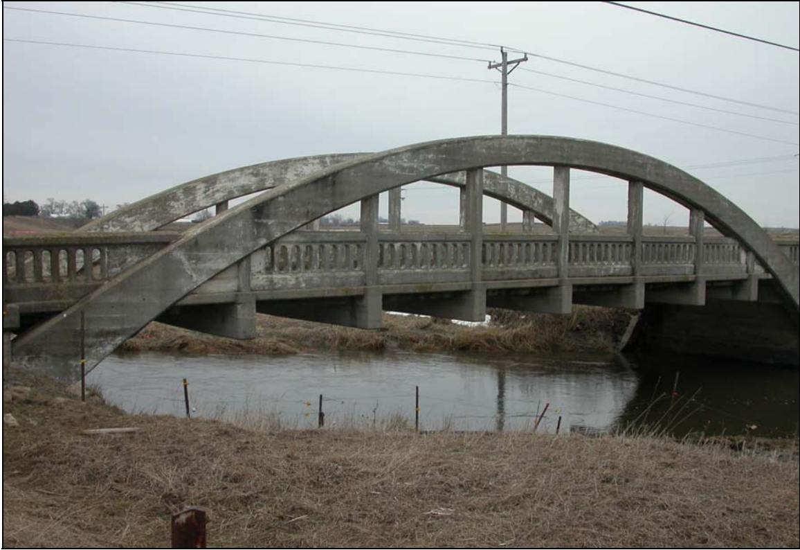
Figure 1. Existing bridge, Boone County
