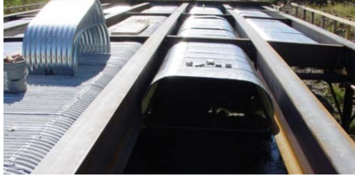
Figure 6. Installed custom-rolled formwork in MBISB 2
