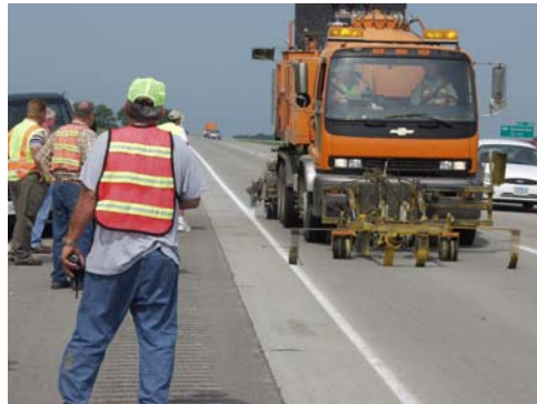
Figure 10. Painting white edge line during the Highways 5 and 65 field demonstration
