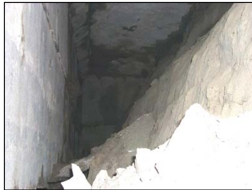
(b) Bridge No. 9703.40020, District 3
