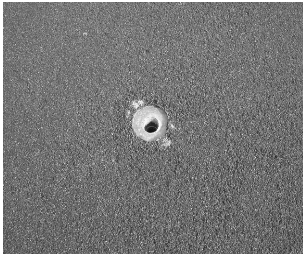
Figure 8. Threaded insert for installation of lifting lugs
