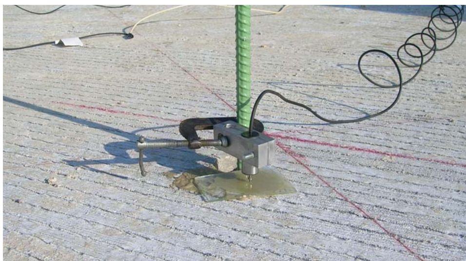
Figure 4. Deflection measurement setup from the first slab
