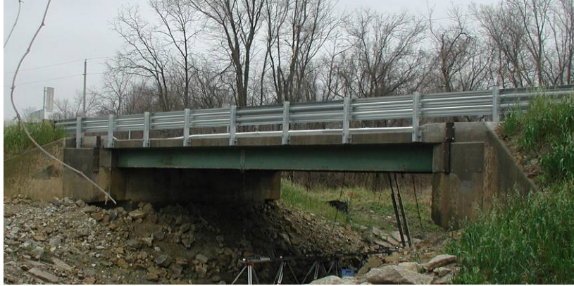
Figure 1. Elevation view of the Tama County bridge
