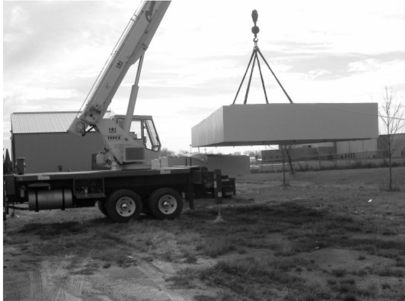
Figure 11. Unloading of individual deck panels
