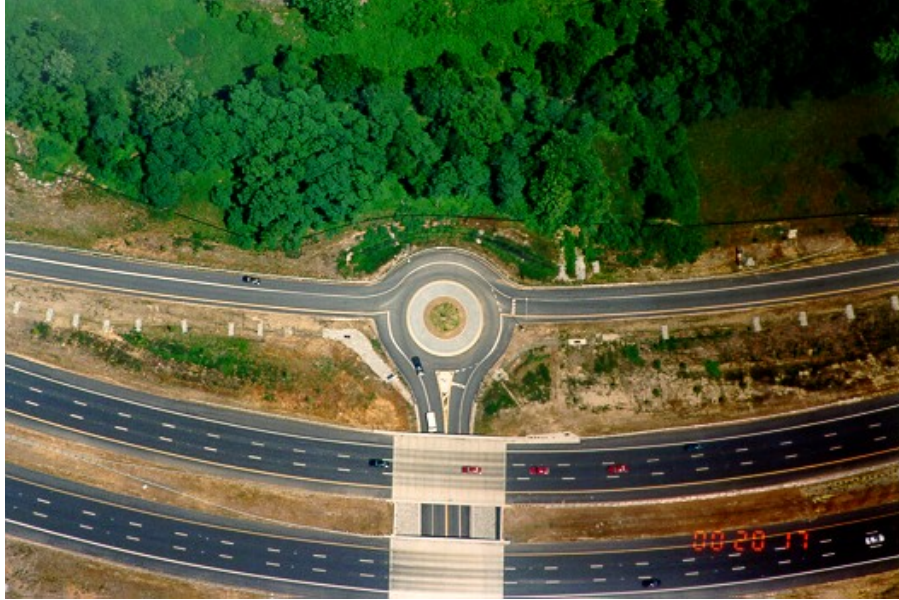
Figure 4. Aerial of MD 100 at Snowden River roundabout
