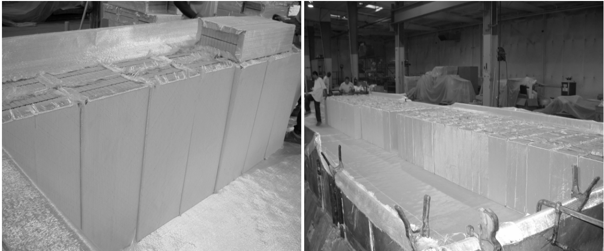
Figure 5. Installation of FRP wrapped foam bottles
