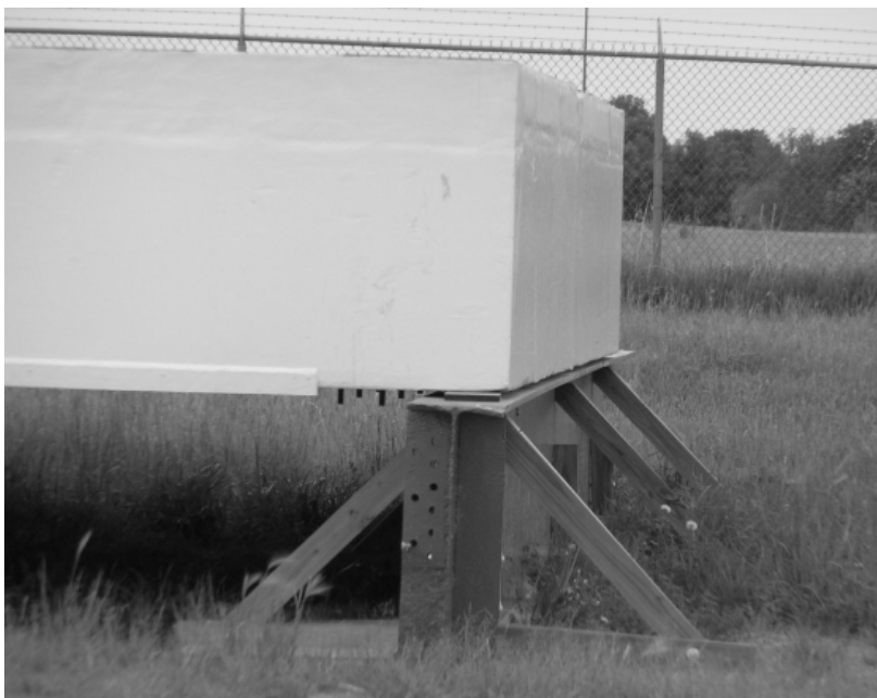
Figure 12. Temporary abutments for Iowa DOT composite bridge
