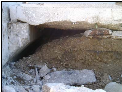
(a) Bridge No. 7779.0065, District 1
