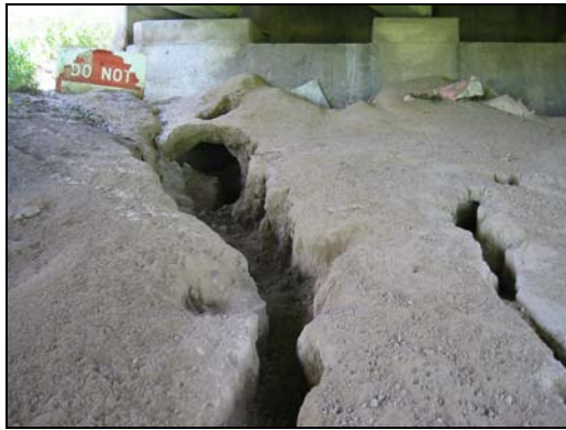
(a) Bridge No. 9703.40020, District 3
