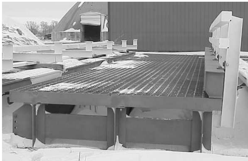
Figure 1. Current steel bypass bridge used by the Iowa DOT
