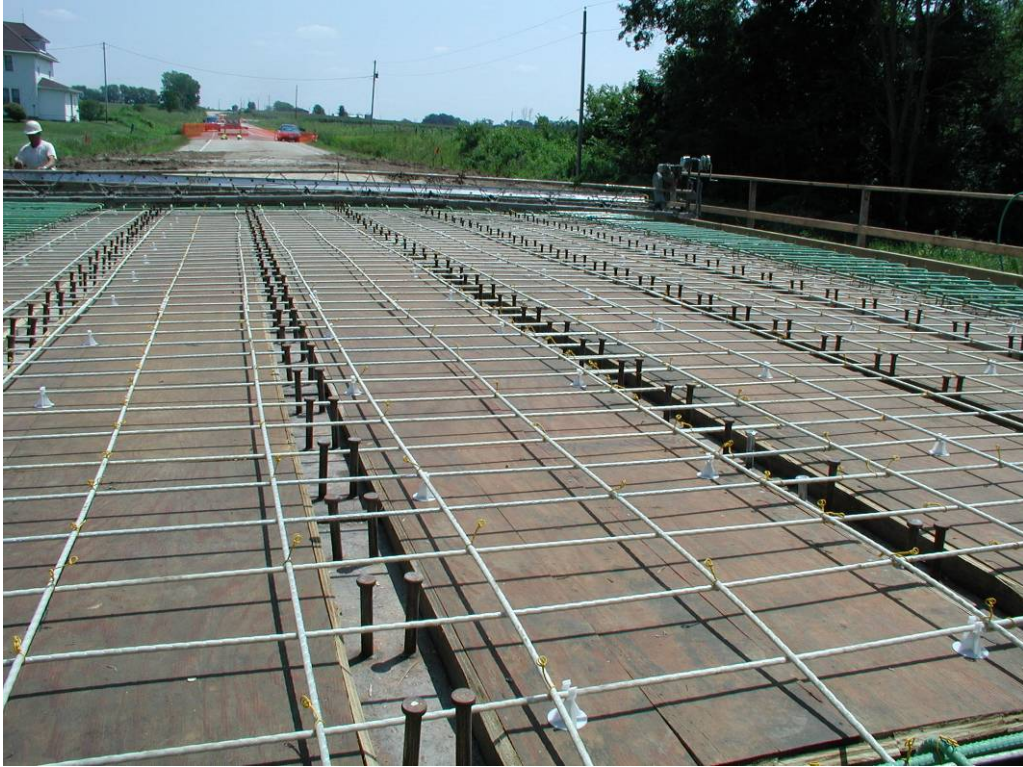
Figure 3. Placement of deck reinforcement
