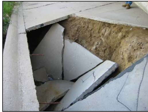
(b) Bridge No. 7871.5L/R029, District 4
