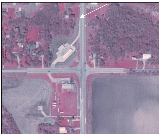
Figure 4. Aerial image signalized expressway intersection
