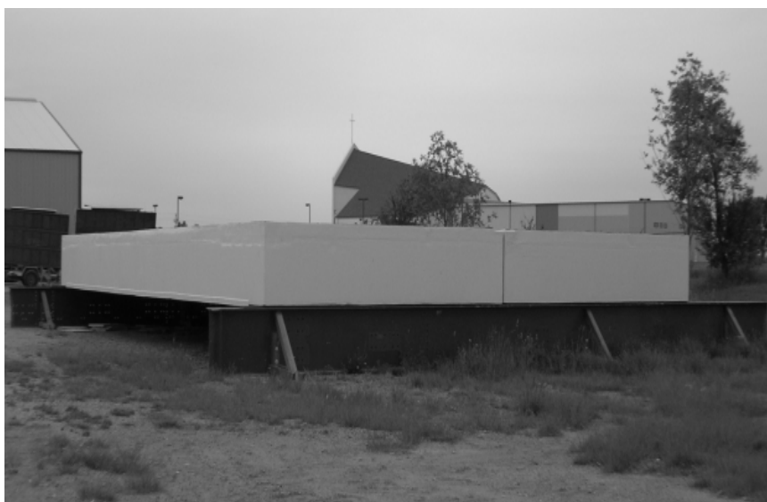
Figure 2. Proposed bypass bridge, w/o guardrail or other hardware, to be used by the Iowa DOT
