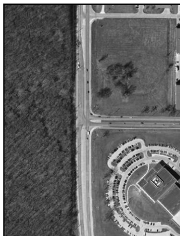
Figure 2. Aerial image of IA 28 and Park Ave
