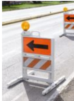
Figure 6. Direction indicator barricade
