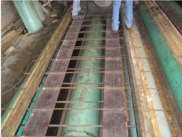
(a) Casting the deck panels
