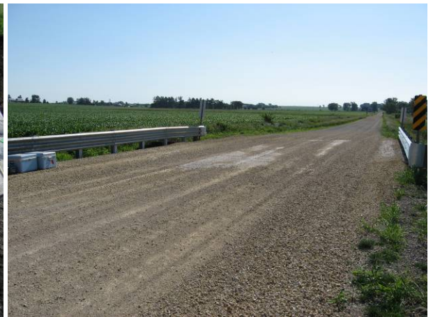
(f) Completed bridge with guardrails
