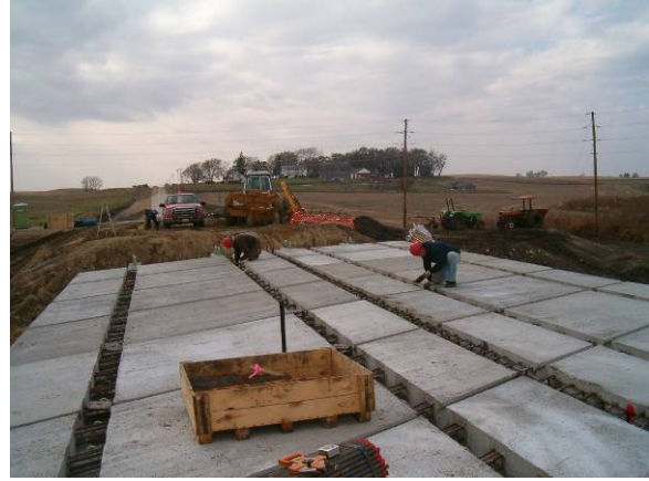
Figure 8. Leveling device installation
