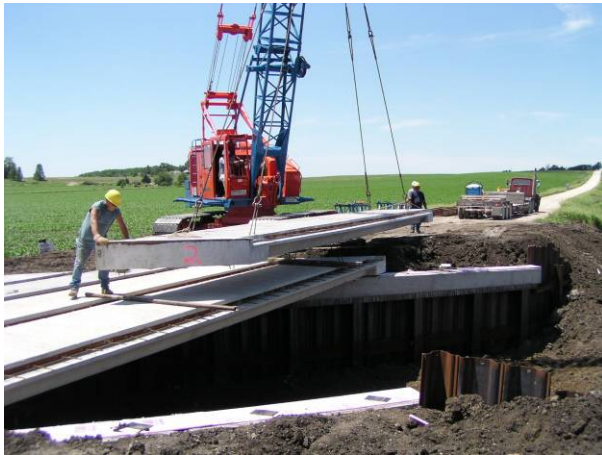
(c) Placing the deck panels
