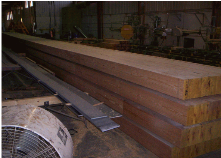
Figure 7. Glued-laminated girders prior to FRP installation
