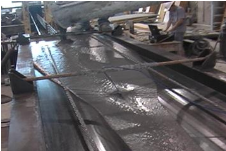
Figure 1. Casting of 110 ft. UHPC beam
