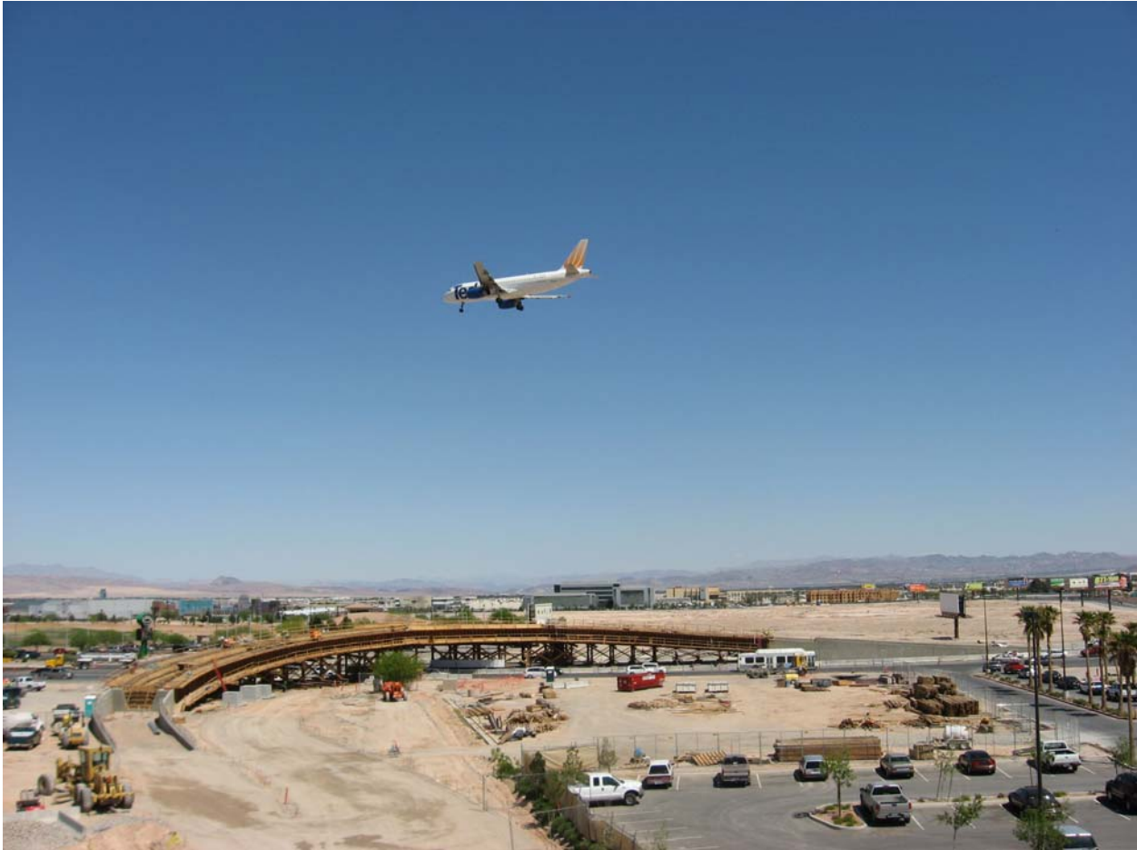
Figure 4. Looking east at the elevated left turn
