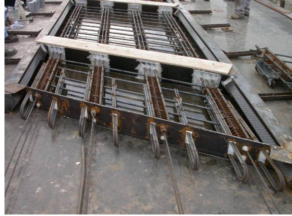
Figure 4. Longitudinal joint reinforcing
