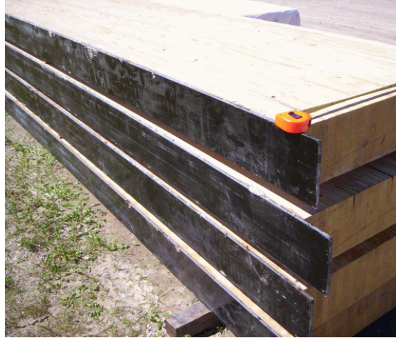
Figure 8. Glued-laminated girders after FRP installation
