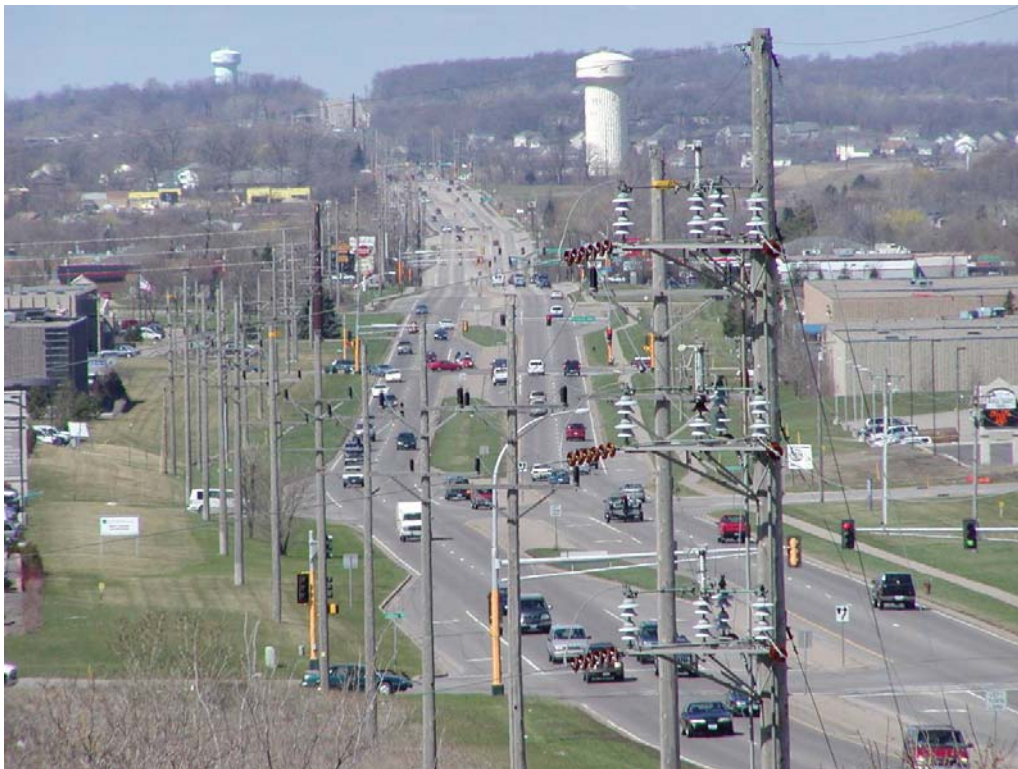
Figure 2. Pre-project view of CSAH 42 looking west (taken by the authors)
