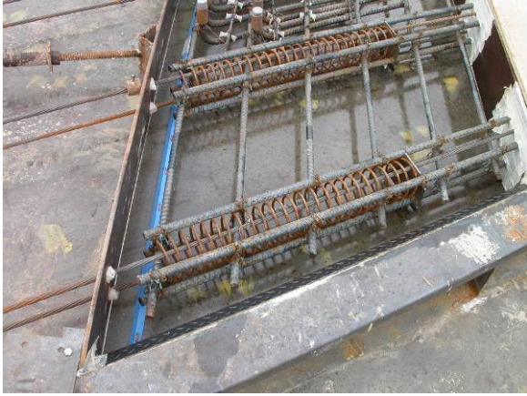
Figure 3. Spiral reinforcing
