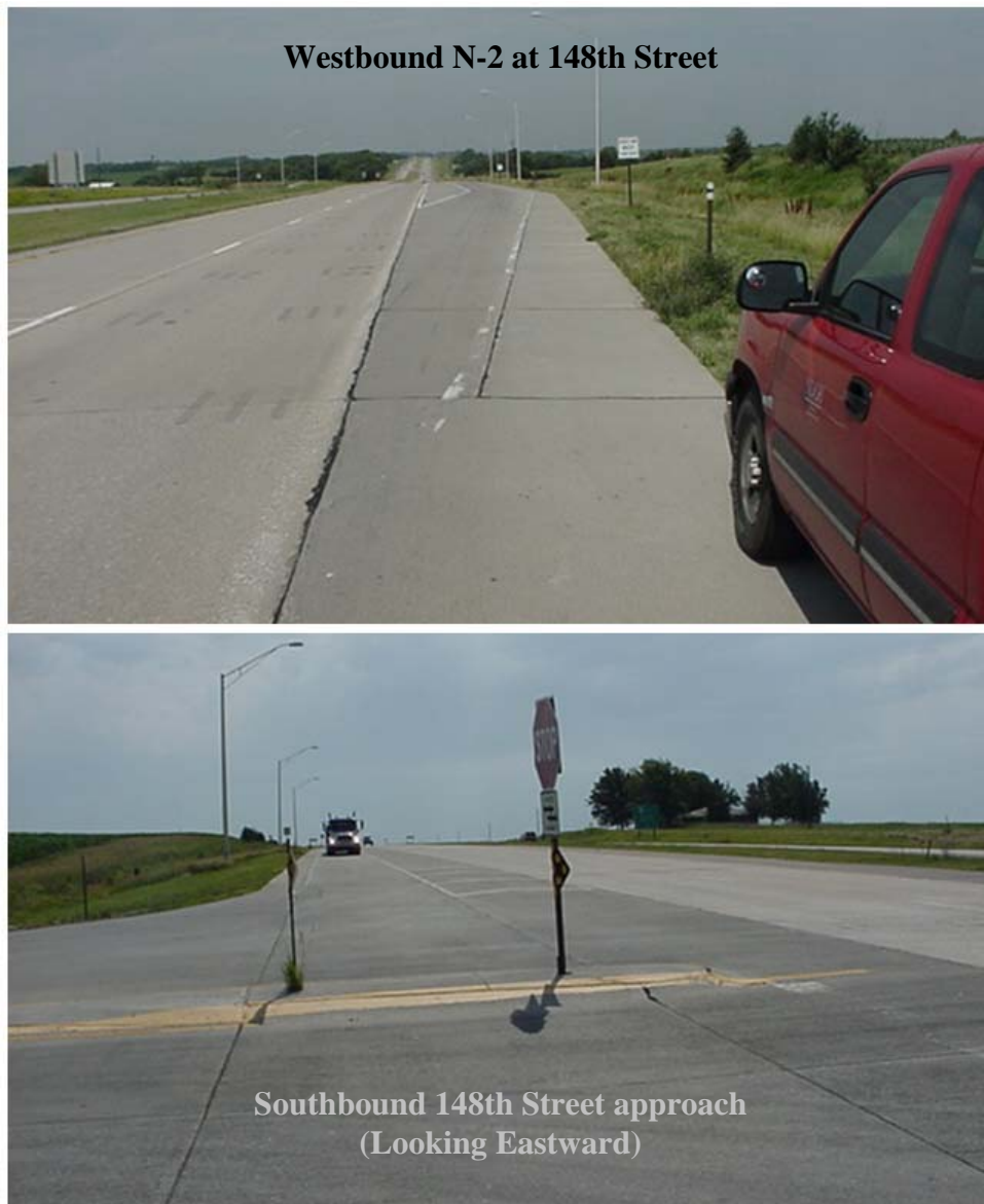
Figure 10. Offset right-turn lane at N-2 and 148th Street, near Lincoln, NE
