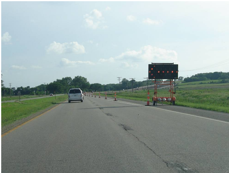
Figure 1. Typical advance warning arrow display at a long-term work zone (arrow displayed)
