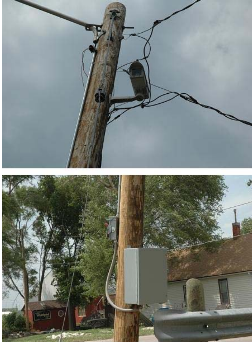
Figure 3. Night vision camera (top) and DVR storage box mounted on a utility pole
