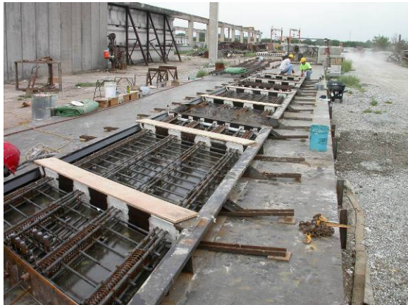
Figure 1. Panel forms and reinforcing
