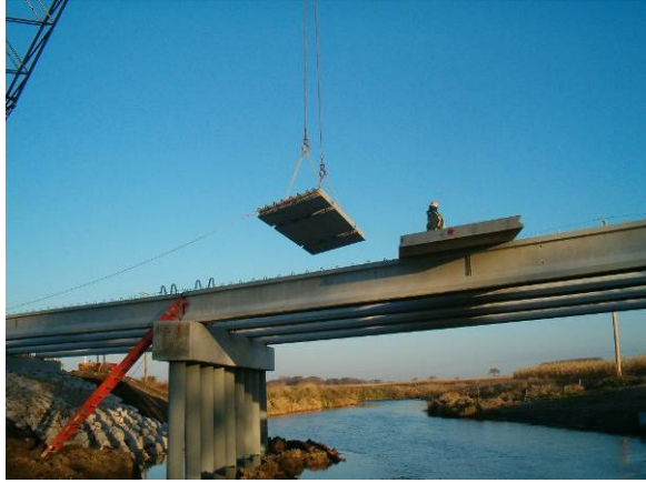
Figure 7. Deck panel erection
