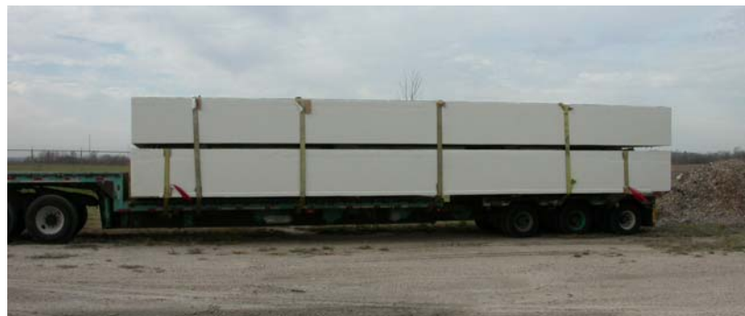
Figure 2. Bridge sections on trailer for transport
