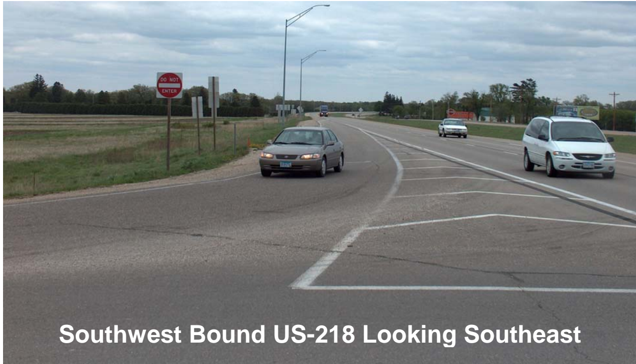
Figure 7. Offset right-turn lane at west junction of US-18 and US-218, Floyd, IA
