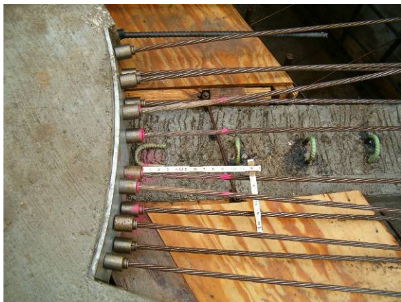
Figure 9. Strand elongation check
