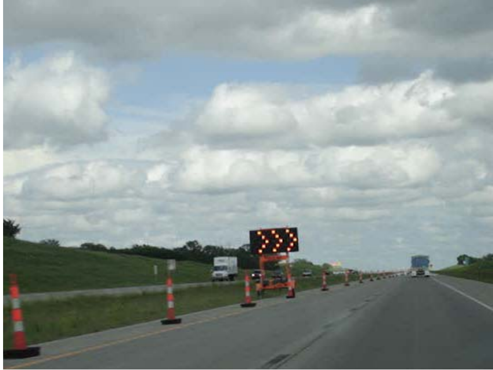
Figure 2. Typical advance warning arrow display at a long-term work zone (chevron displayed)
