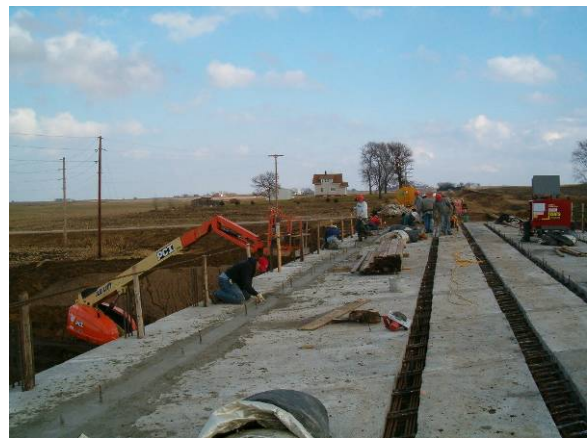
Figure 10. Casting longitudinal joints
