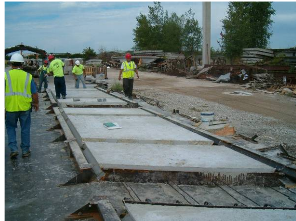
Figure 2. Panel form release
