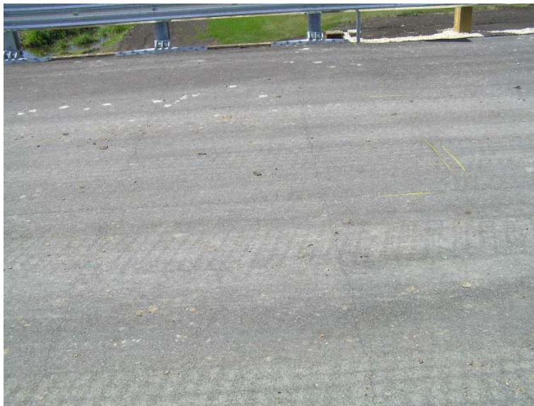
Figure 3. Delaware County Bridge wearing surface
