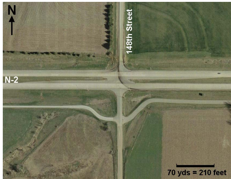
Figure 9. Intersection of N-2 and 148th Street, near Lincoln, NE
