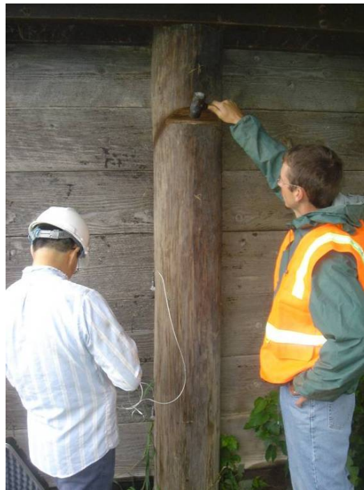
Figure 3. Pile integrity testing (Bridge No. 237350, Mahaska County)
