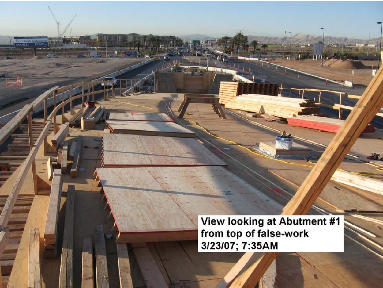
Figure 1. View looking at abutment #1 from top of falsework
