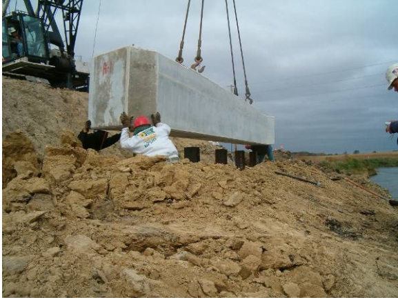
Figure 5. Setting precast abutment
