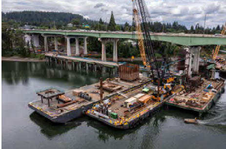
Construction barges on the Willamette River looking into West Linn.
