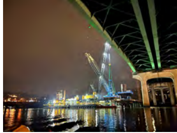
Nighttime construction work on the river.
