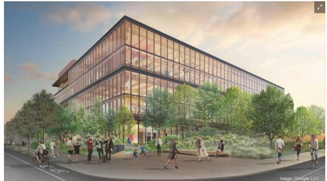
Google has begun construction of its first mass-timber building in Sunnyvale. The five-story project could pave the way for future buildings constructed using that method.
