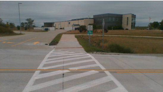
WORKING WITH KIRKWOOD COMMUNITY COLLEGE AND ADA RAMPS
