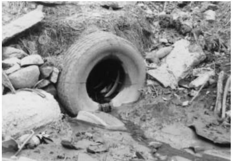
*Not only do truck tire culverts save money, but these drainage structures represent a significant reuse of scrap tires.*
