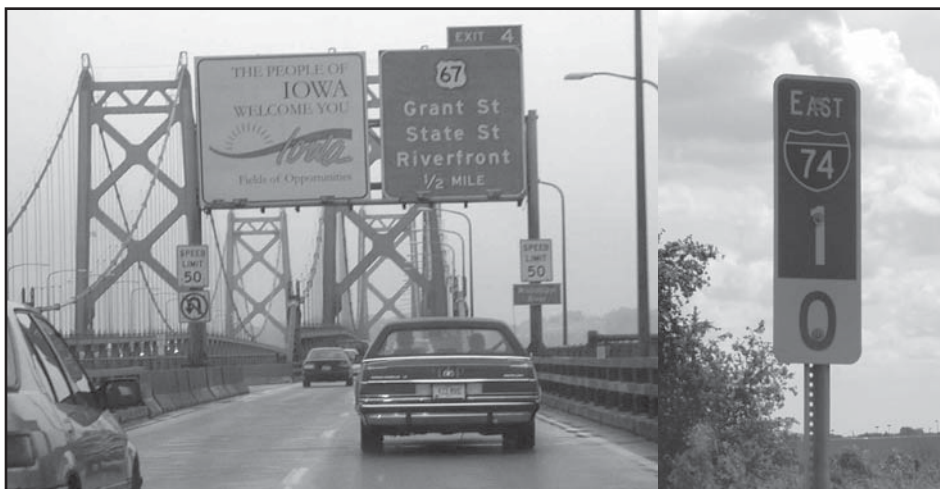
CARS improved safety on the I-74 bridge by installing one-tenth mile markers for motorists to identify their location in case of a crash, dynamic message signs to warn approaching motorists of delays due to crash, and cameras to help law enforcement monitor crash sites and traffic backups.
