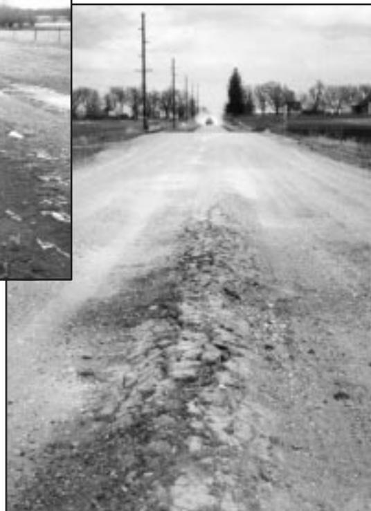
Poor drainage causes water to seep into the roadbed and cause problems like this frost boil (right).
