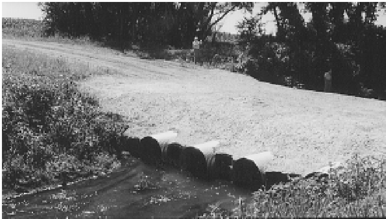
Vented ford with pipes (Tama County, Iowa)
