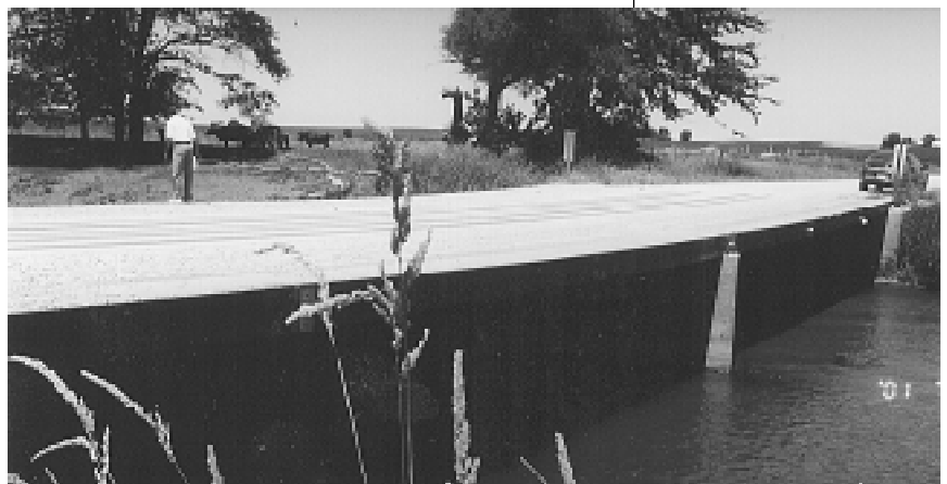
Low water bridge (Benton County, Iowa)
