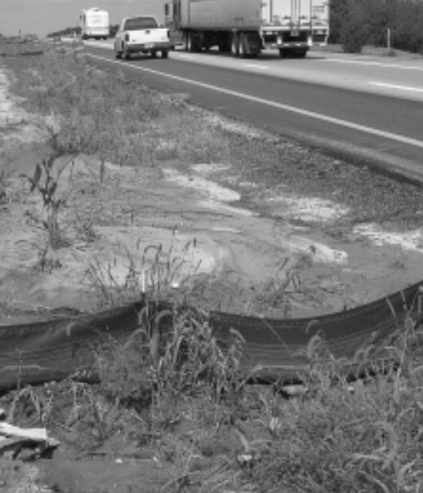
A silt fence is placed near a slope drain to prevent soil and silt from washing down the right of way.
