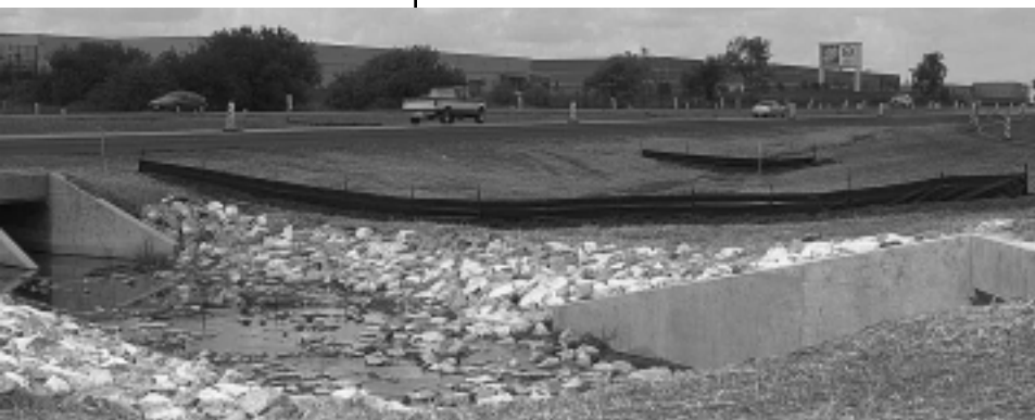
This picture shows two different types of erosion control: stones lining the bank of a waterway and silt fences in the road's right of way to hold soil and silt in place.
