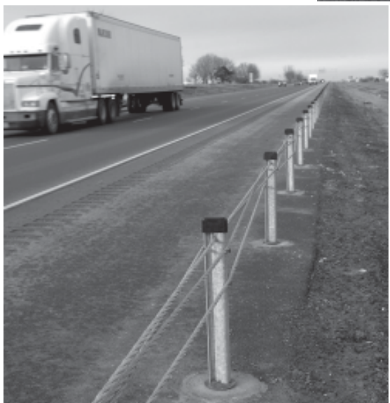
Four cables absorb energy from an impact. Photos courtesy of the Iowa DOT.
