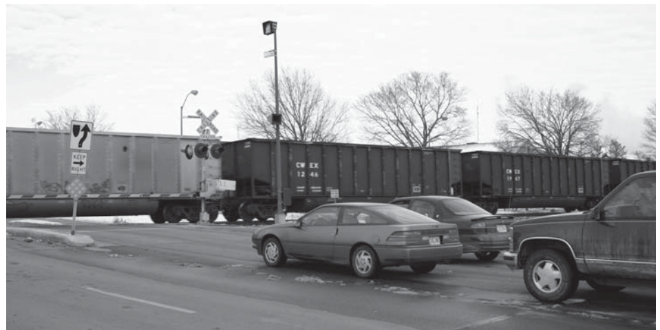
Having gates and lights at a railroad crossing is not enough to qualify that crossing for a quiet zone.
