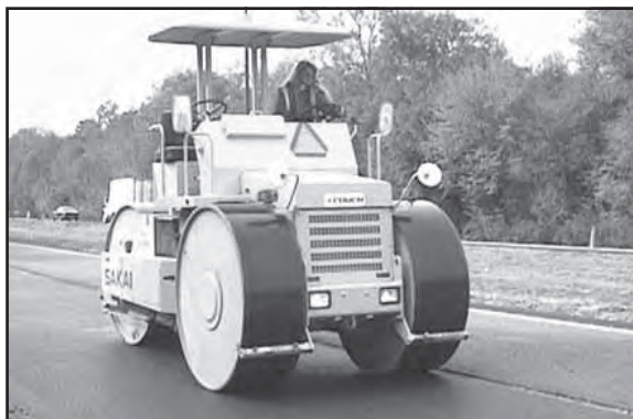
A consistent roller pattern helps achieve density, an important quality for hot mix asphalt longevity. Photo courtesy of the National Center for Asphalt Technology.
